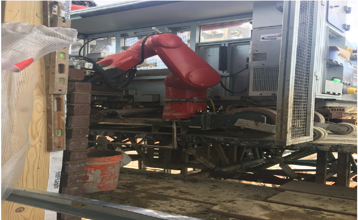
Brick being installed by SAM: Semi Automated Mason
