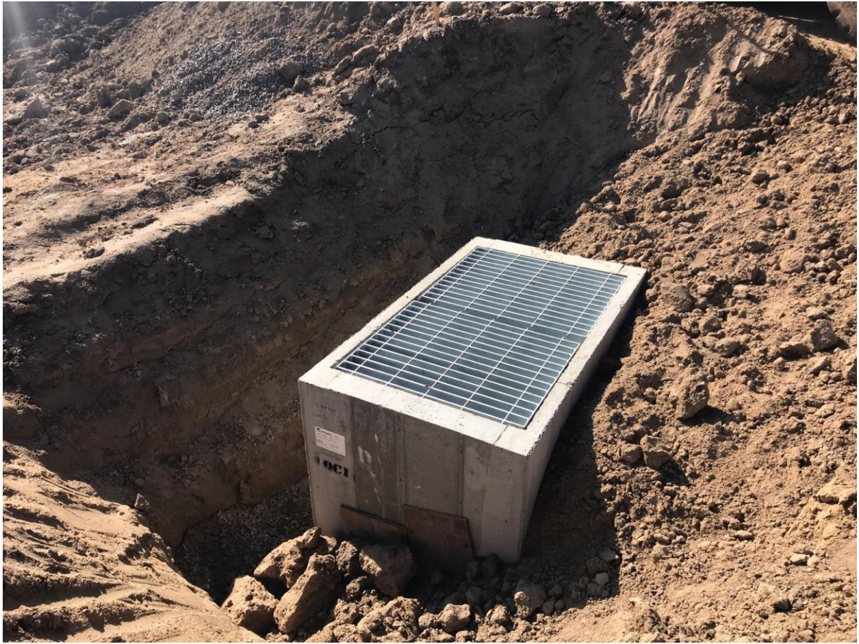
Storm Vault Installed (SW Corner of West Side)
