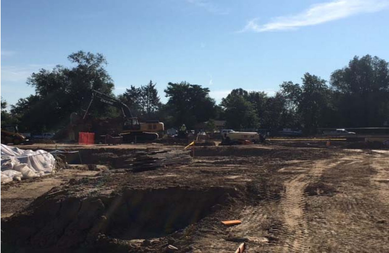
Photo from center of site, looking northeast.
