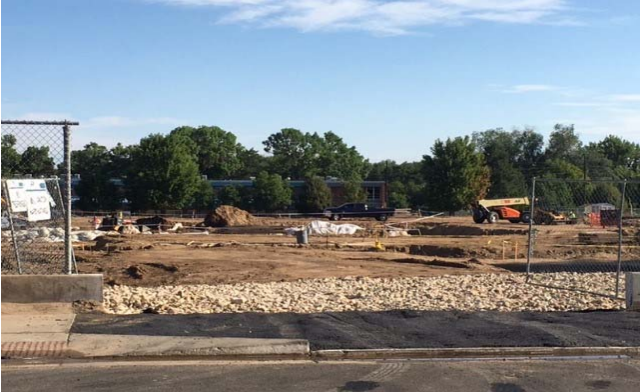
Photo from Union at construction entrance, looking north.
