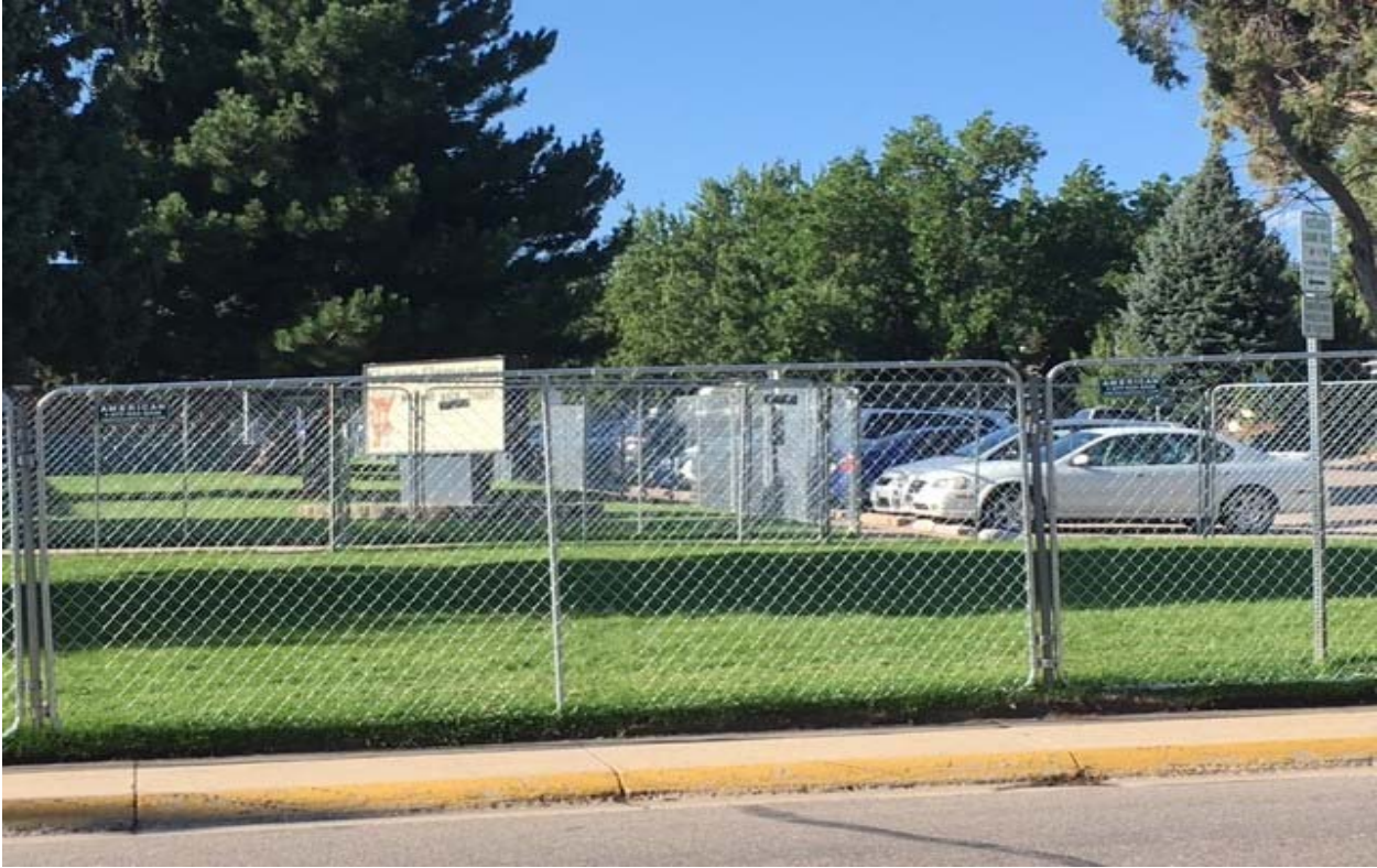
Safety fences for recess areas are installed.
