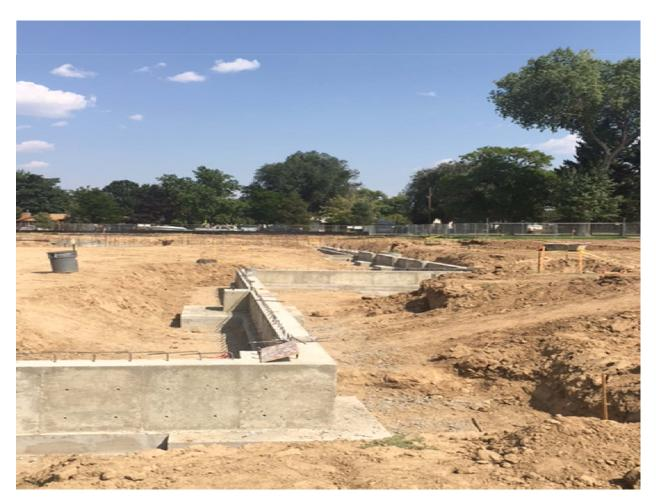
Walls being formed for concrete pours next week for NE, north and NW corner
