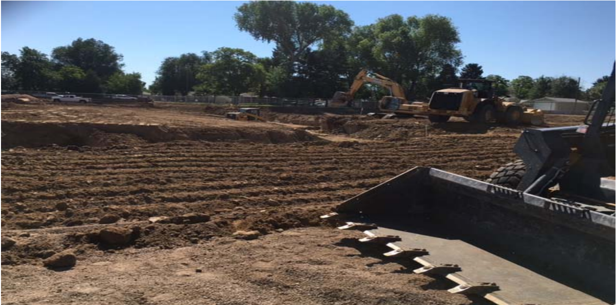
Photo taken from center of the site, looking southeast.
