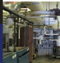
**HVAC:** Aging system of univents, RTUs and some baseboard heat. Univents are noisy and create a barrier to learning. The school has one boiler room containing four boilers. All four are over 25 years old. Control systems are out of date. Much of the electric service is in excess of 15 years old. Several new circuits have been added to accommodate new technology and equipment.
