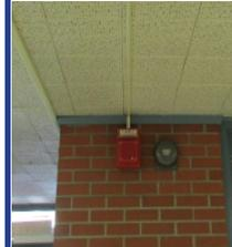
**Safety Devices:** Fire alarm system is over 15 years old and does not meet current fire code. No fire sprinkler system in the building. Building is equipped with a functioning alarm system containing door contacts and motion sensors. The system is out of date. Building has buzz-in intercom with security camera for entry. No security vestibule. Analog intercom system installed in 2008.
