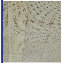
**Building Structure:** Gym and library roofs were replaced in 2015. All other roof sections are in excess of 15 years old. No persistent leaks noted. Evaporative coolers create excess humidity in the space, which has caused the ceiling tile adhesive to fail in some cases. No noted exterior wall issues and no noted foundation issues.
