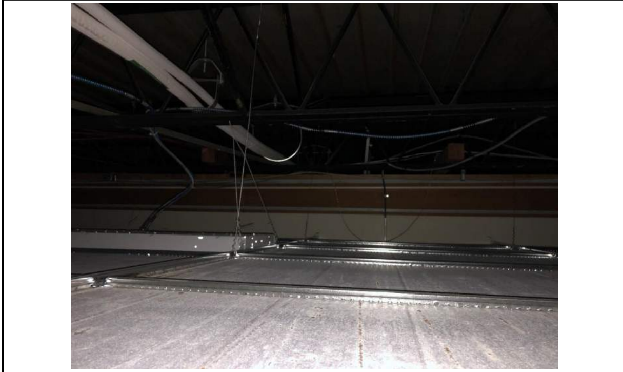
Photo Number: 2 Location: Above ceiling, Classroom 10 Date: December 23, 2019
