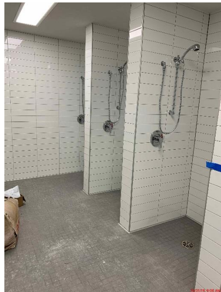
Progress Photo: SFHS Girls locker room showers tiled
