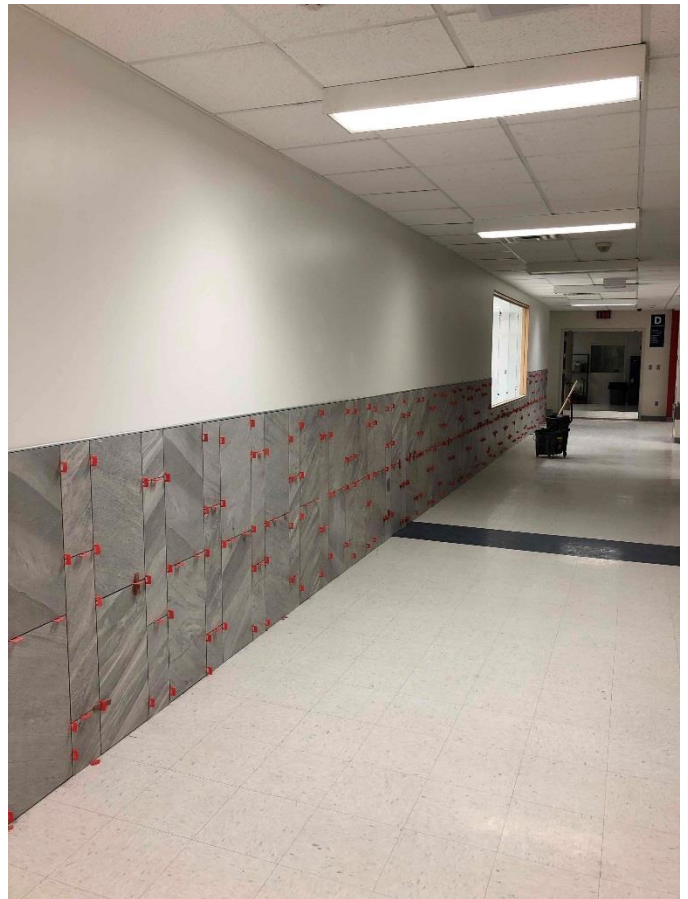
Progress Photo: SFHS Tiling going up on wall in area L
