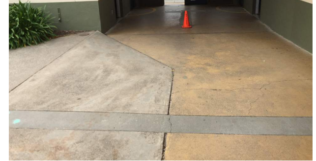
Typical Concrete Paving
