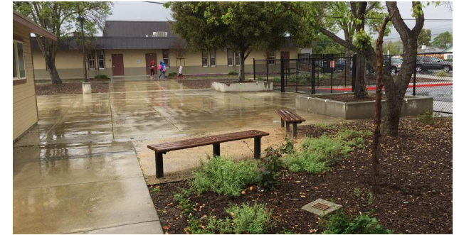
Typical Concrete Paving
