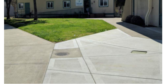
Typical Concrete Paving
