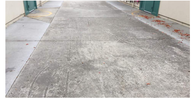
Typical Concrete Paving
