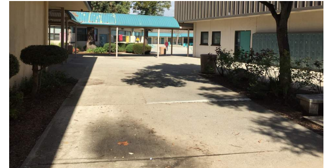
Typical Concrete Paving
