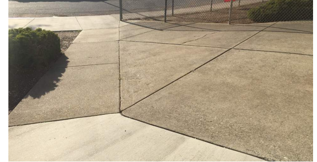
Typical Concrete Paving
