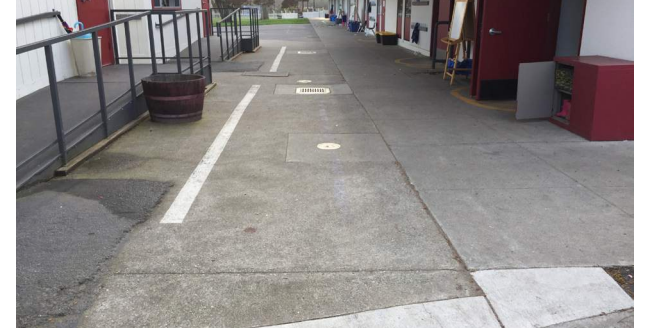
Typical Concrete Paving
