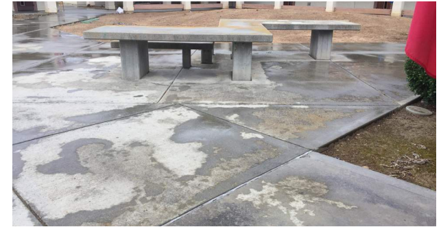
Typical Concrete Paving
