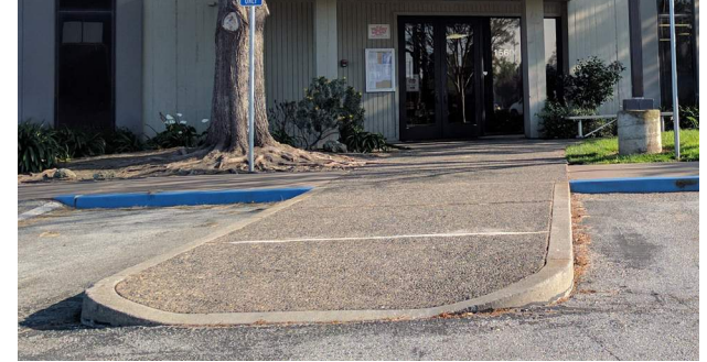
Typical Concrete Paving
