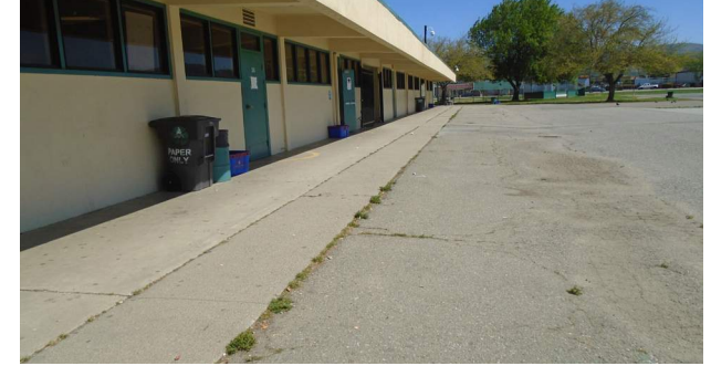
Typical Concrete Paving
