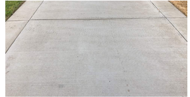
Typical Concrete Paving
