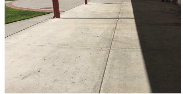
Typical Concrete Paving
