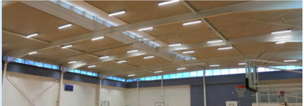
Energy efficient lighting
