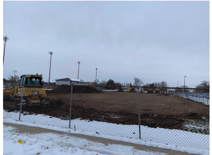
Above: Existing upper practice field on the site was stripped of topsoil last week. This area will become parking lot and expand on
