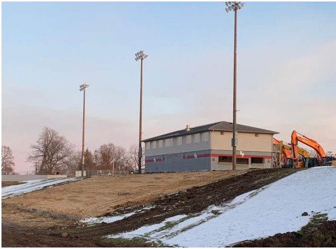
Above: The existing bleachers & concrete foundations were removed.
