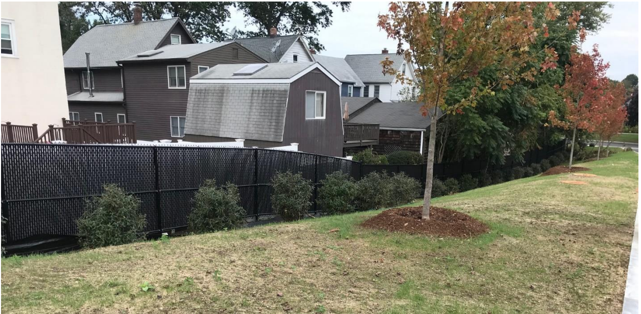
Privacy Fence installed along property line - 10/2/19
