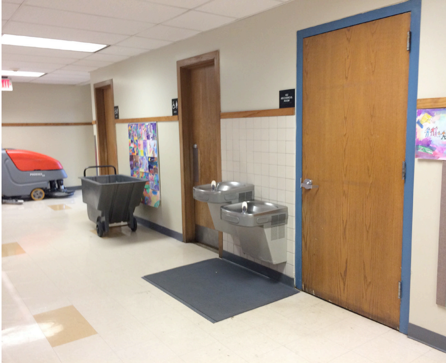
Drinking fountains protruding into Corridors more than allowed by ADA.
