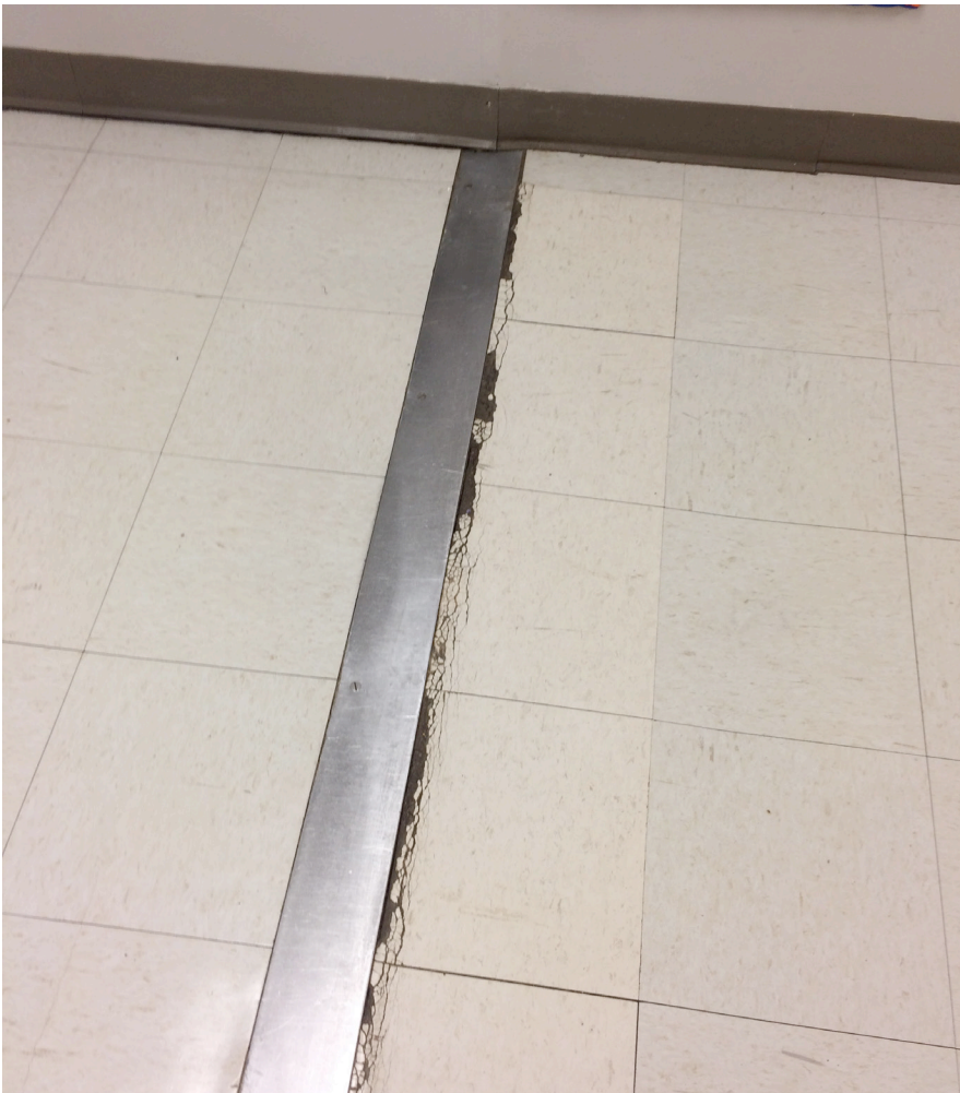
VCT flooring with cracks at expansion joints. There are also uneven surfaces at walls and ceilings. VCT flooring is a maintenance issue.
