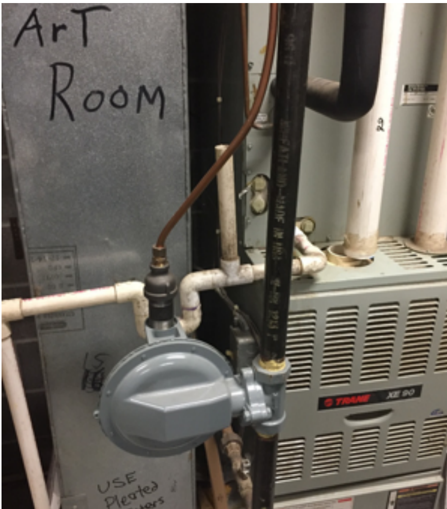
Split system serving Art Classroom. Exhaust not connected to unit.
