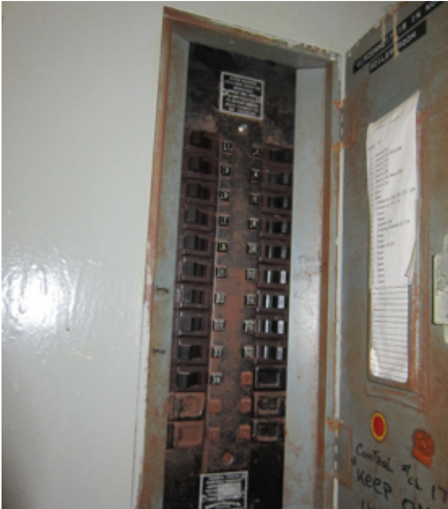
Old electrical panel with significant amount of rust
