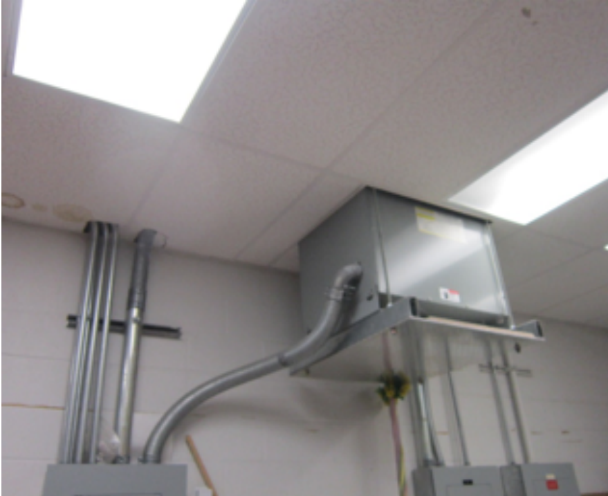
Electrical Transformer with Limited access due to ceiling installation
