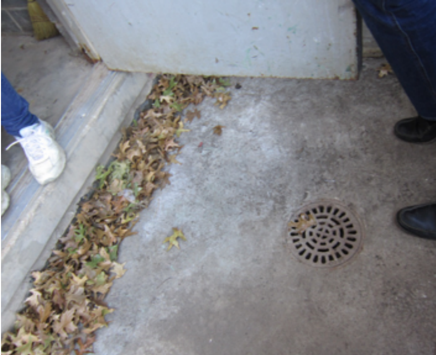
Exterior drain at mechanical room that clogs easily causing water inside building
