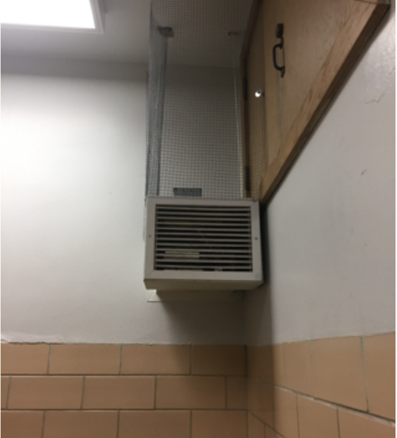
Transfer air from restroom to corridor.
