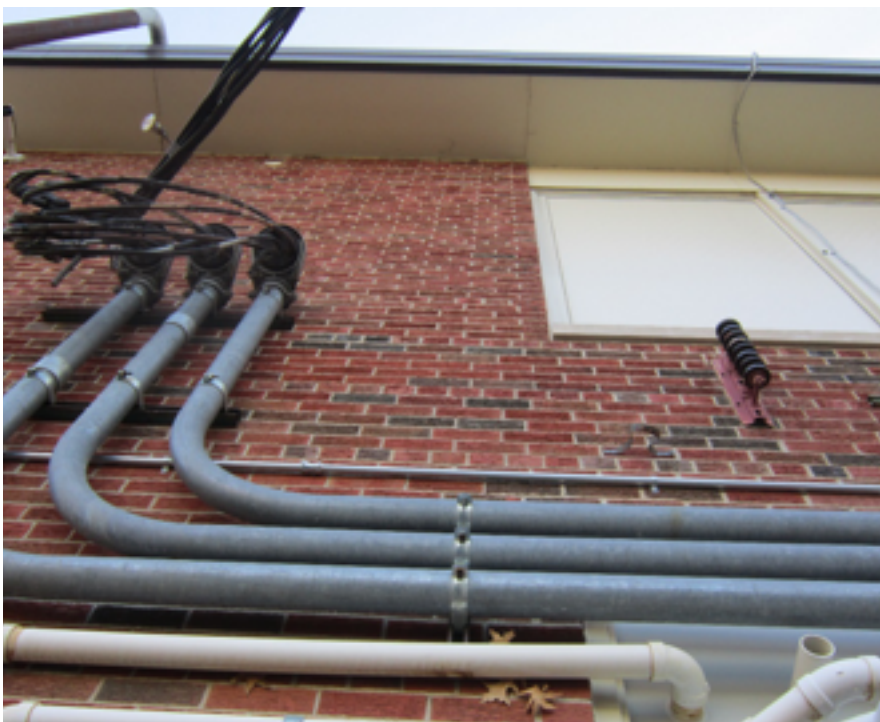
Overhead Electrical Service
