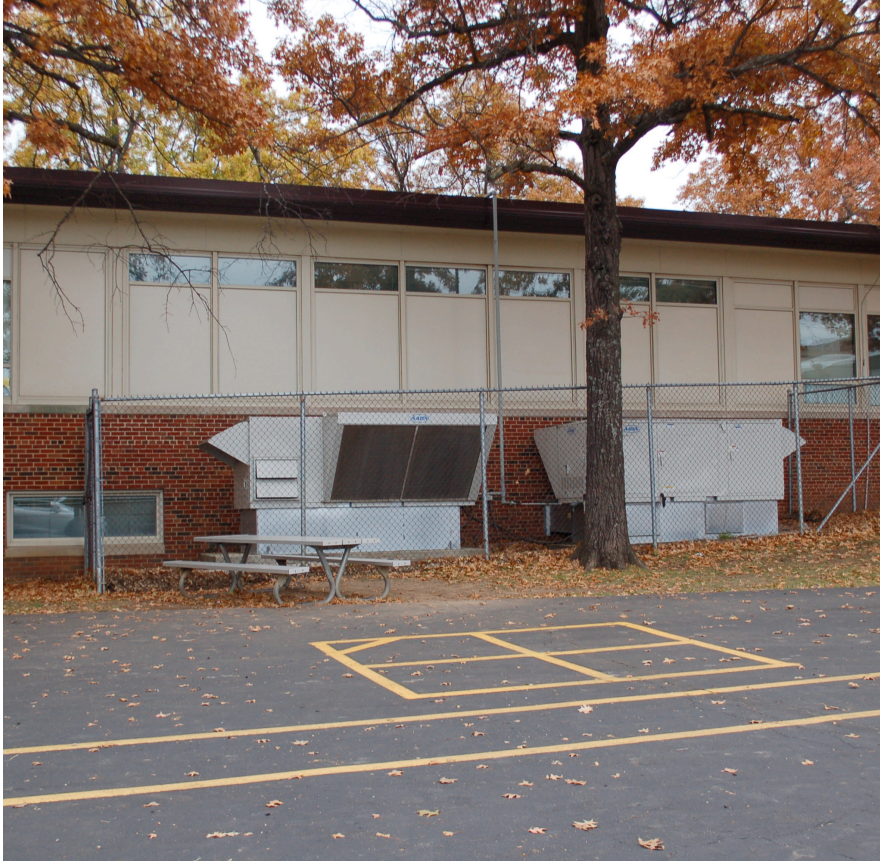
Noisy HVAC exterior unit adjacent to classroom windows.
