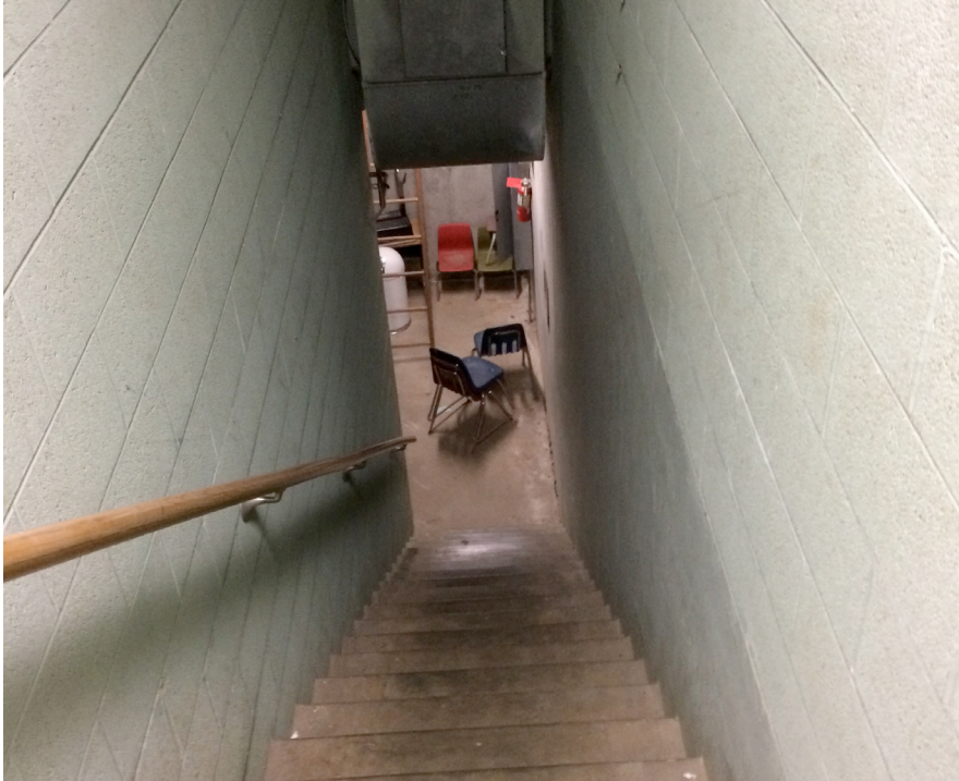
Steps to basement mechanical room too steep (7 \frac{3}{4} " risers and 10" treads)
