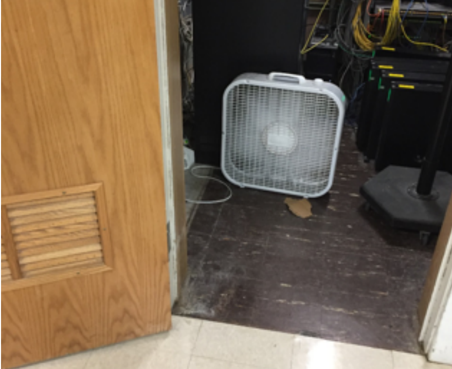
Cooling for data closet is a portable fan with louver in door
