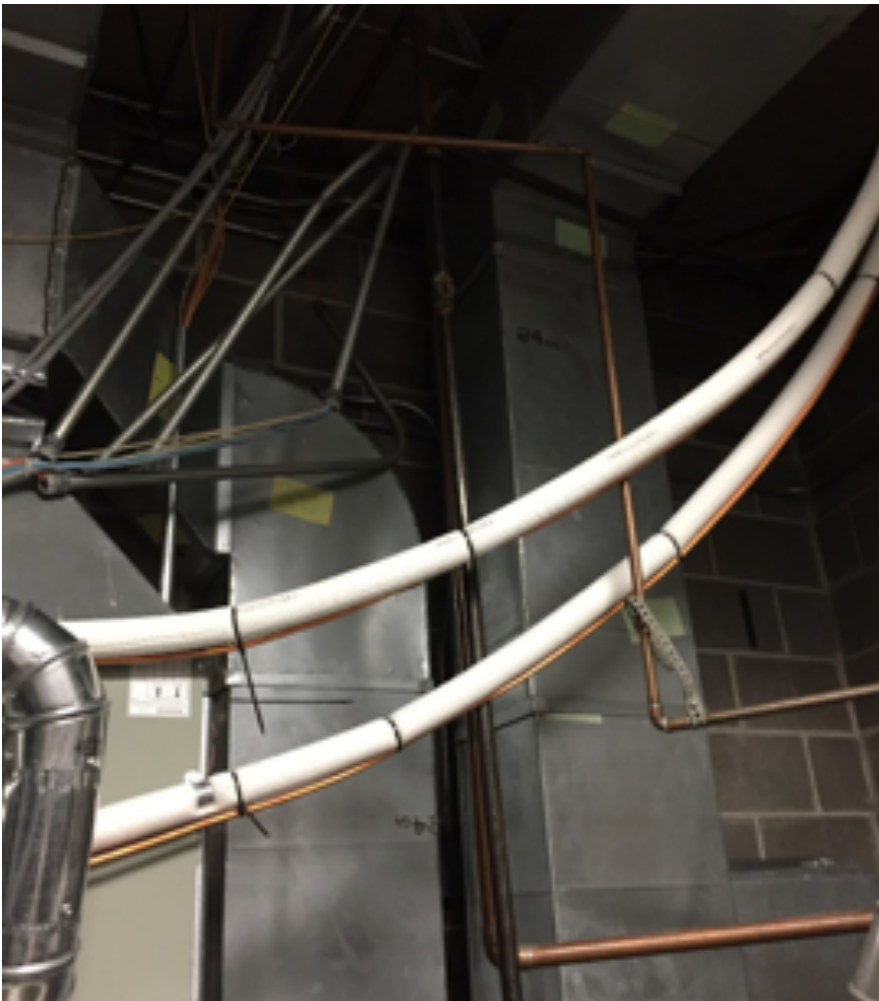
Domestic water piping not insulated
