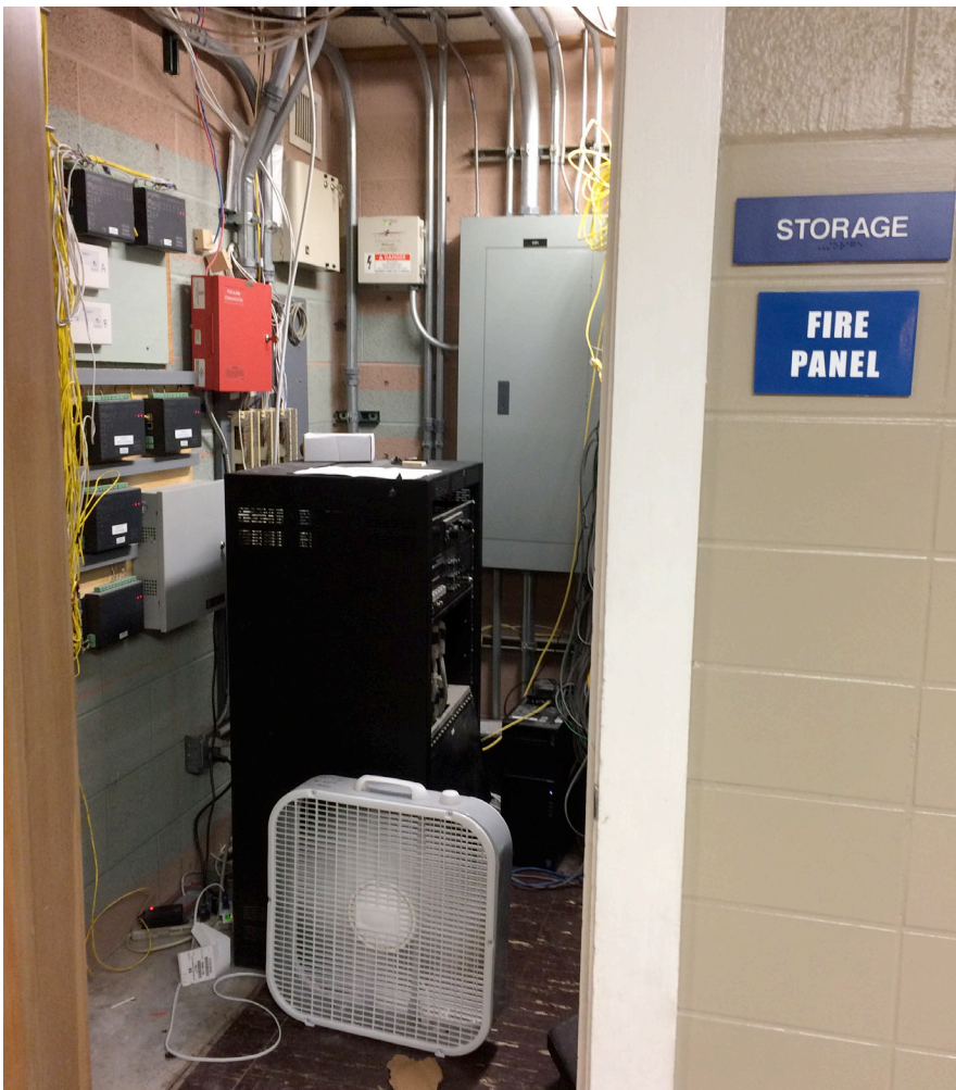
Fire Panel room has equipment that require a cooler space. The box fan is not adequate.
