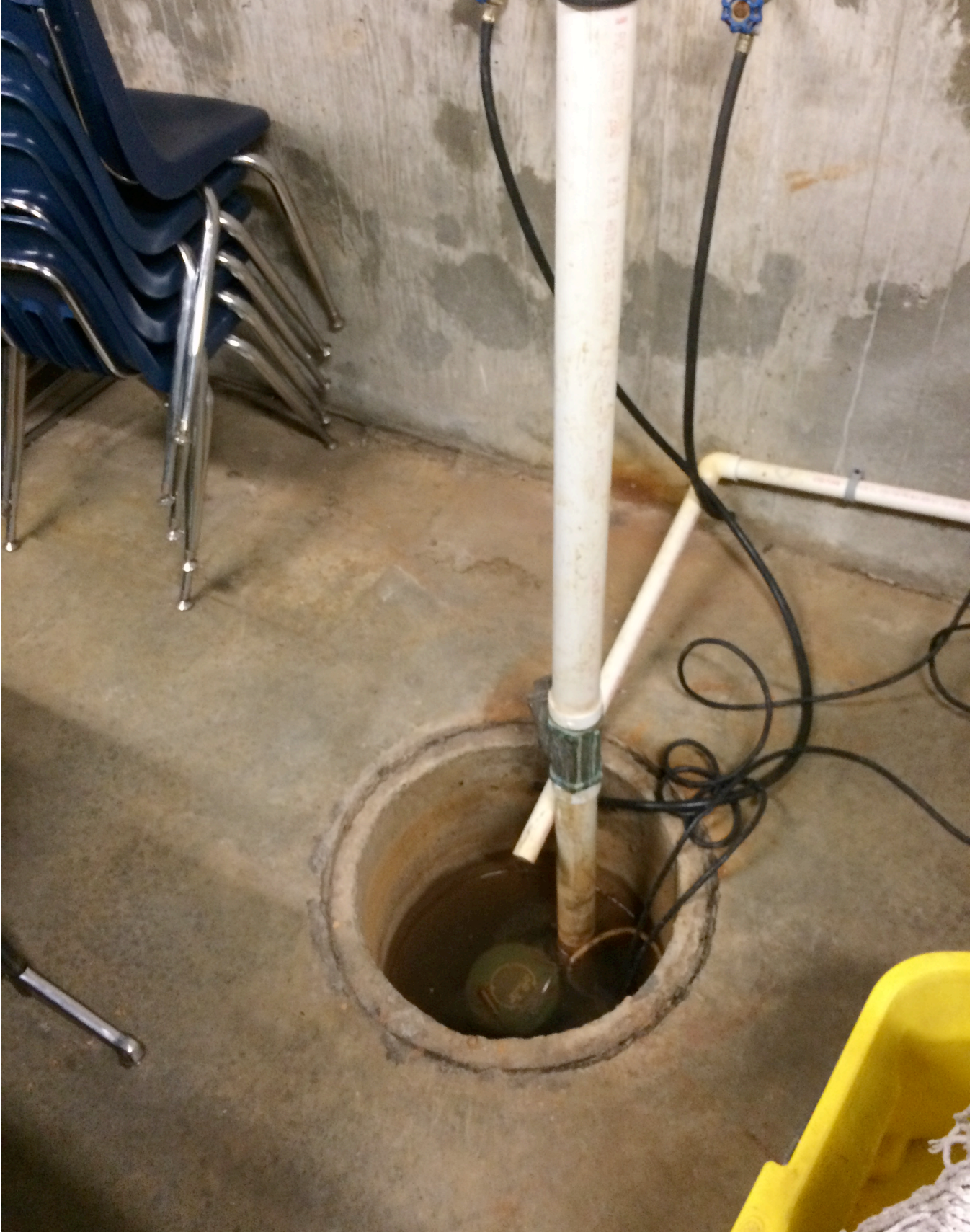
Broken sump pump at Basement Mechanical Room.
