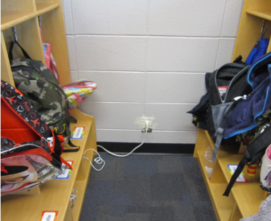
Electrical cord secured in place with tape
