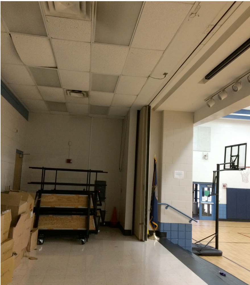
Stage: Droopy ceiling tiles as a result of humidity issue. Accordion door is used at stage to create a separate room when needed, but the acoustics are bad so the room is not used for a classroom.
