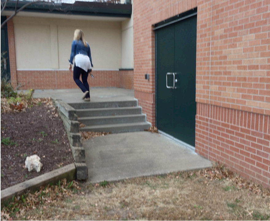
Water from the adjacent low roof dumps rain water in front of gym doors and water drains into the gym. Sidewalk outside gym doors needs an area drain.
