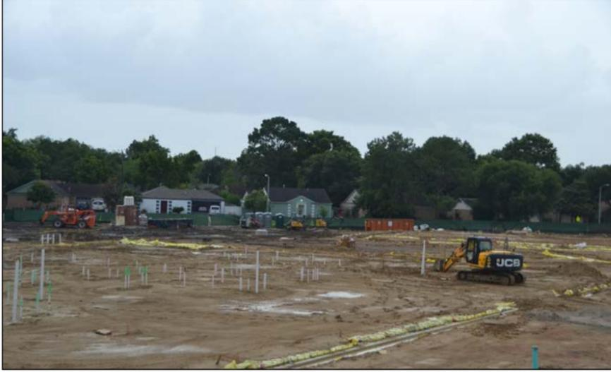
Plumbing has been installed and grade beams have been poured in preparation for the slab at the new Baker Sixth Grade Campus facility, which will be located south of the Instructional Technology Center on the current Baker campus.
