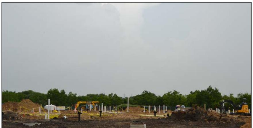
The construction team prepares to pour the slab at the new Lomax Elementary School, where plumbing has been installed and grade beams have been poured. The new Lomax facility is being built on the northeast corner of the current site.
