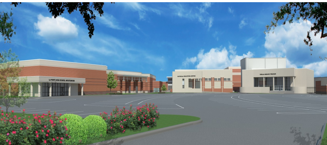
View of Natatorium Building
