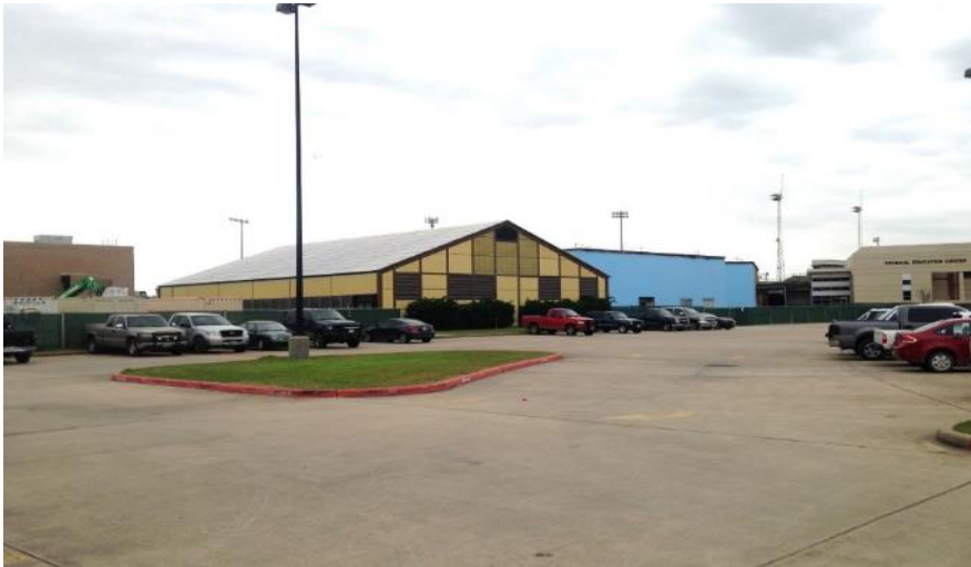
Site of New Natatorium – “Before”
