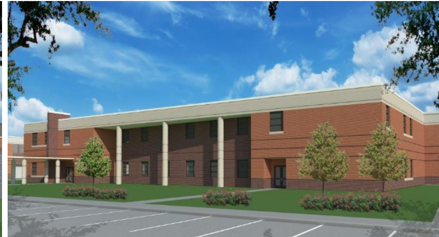
View of Math and Science Building
