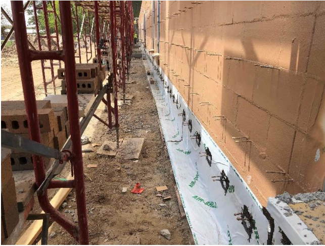
Progress Photo: EBES weather barrier progress.
