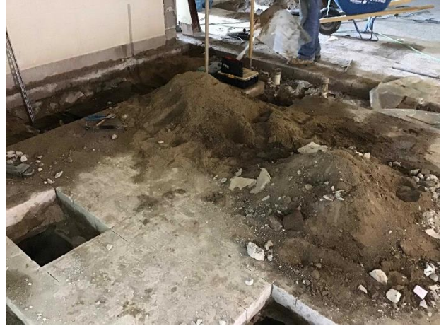
Progress Photo: SFMS Area A kitchen demo progress.
