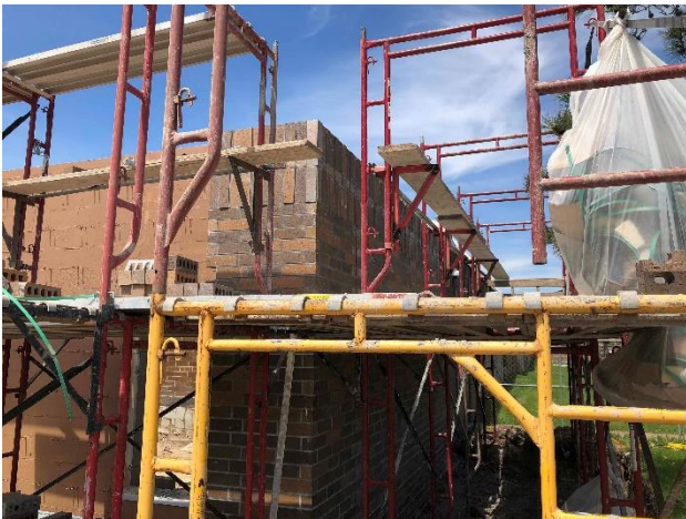
Progress Photo: EBES classroom addition exterior wall brick progress.
