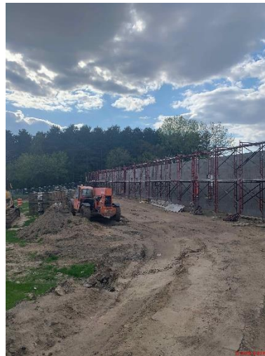
Progress Photo: EBES Classroom addition pre weather barrier.
