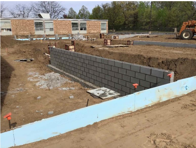
Progress Photo: SFES Classroom addition foundation wall progress
