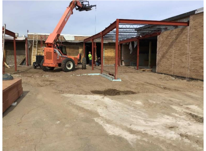
Progress Photo: SFES bus entry addition structural steel.
