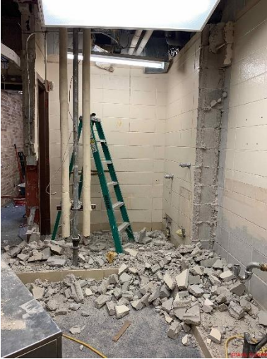
Progress Photo: SFES Area B Demo
