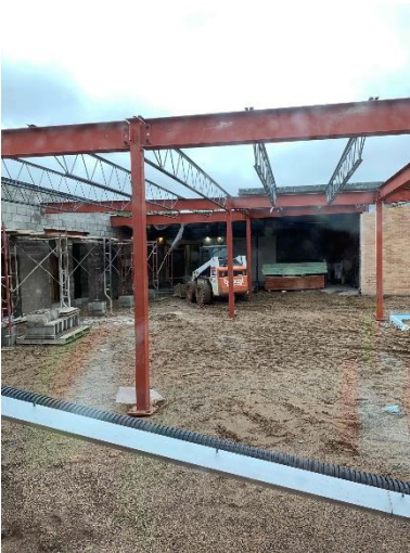
Progress Photo: SFES East side entry addition structural steel progress.
