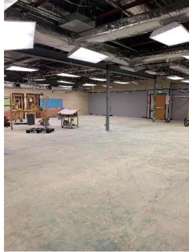
Progress Photo: SFES Media Center demo progress.
