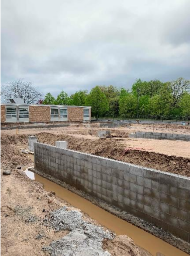
Progress Photo: SFES Classroom addition foundation wall progress.
