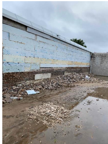
Progress Photo: EBES Classroom addition exterior wall demolition.
