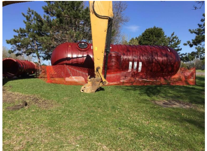
Progress Photo: EBES Fire protection water tank
