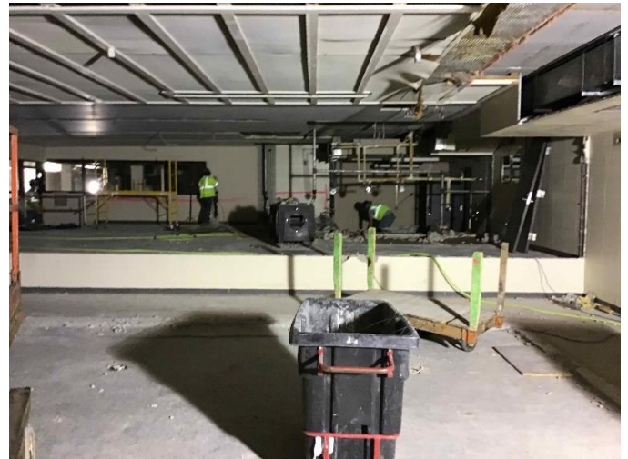
Progress Photo: SFHS Locker room demo
