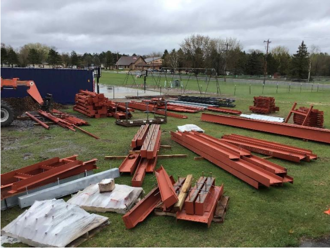
Progress Photo: SFES Structural steel
