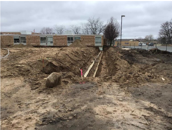
Progress Photo: SFES Classroom addition footings
