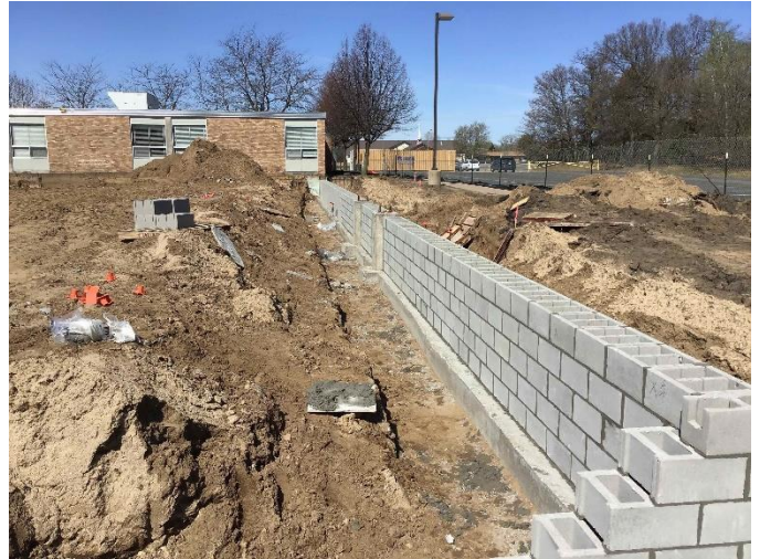
Progress Photo: SFES classroom addition foundation wall
