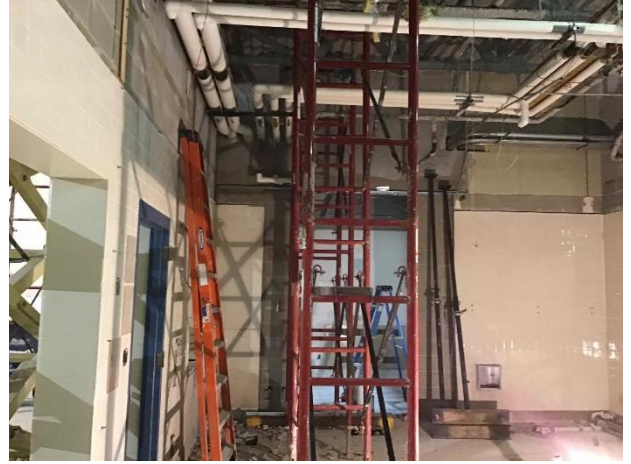
Progress Photo: SFMS kitchen demo area A
