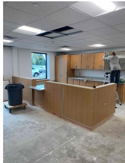
Progress Photo: EBES Area B reception desk
