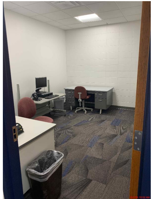
Progress Photo: SFMS Area E SPED flooring install
