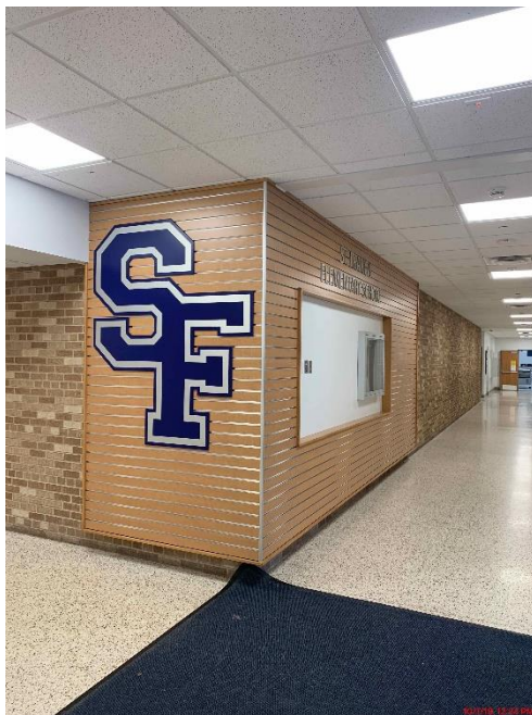
Progress Photo: SFES School branding wall
