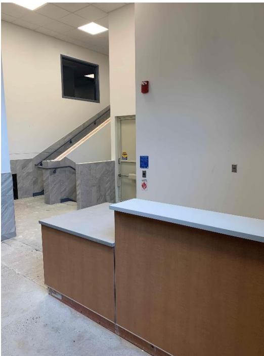
Progress Photo: SFHS Area H greeter station
