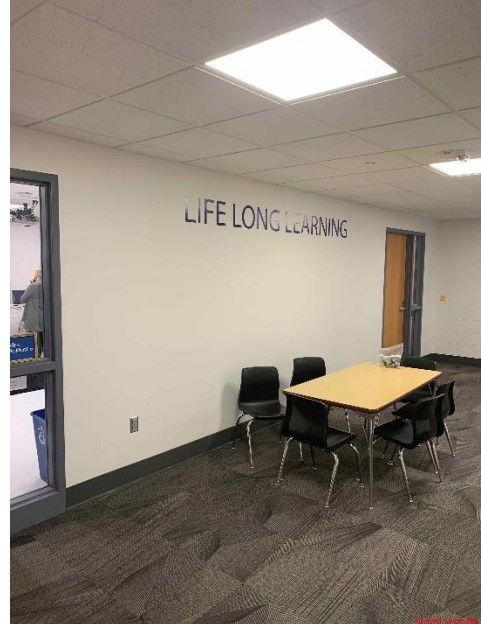
Progress Photo: SFES Area D SPED resource area
