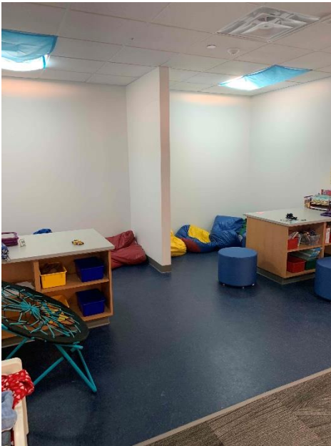
Progress Photo: EBES Area C SPED resource area
