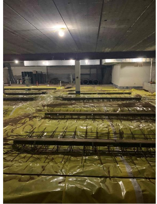
Progress Photo: SFHS Area C locker room progress
