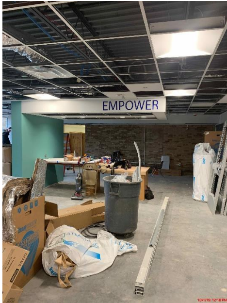
Progress Photo: SFES Area D open media Center
