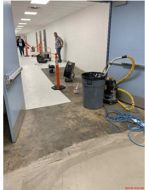
Progress Photo: SFMS Area E hallway flooring install
