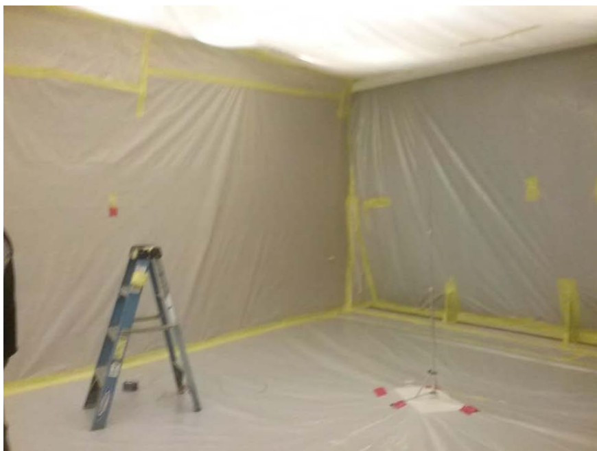
Photo 14 Depicting Ambient Sample Apparatus in Upper North area following installation of enclosure isolating walls, ceiling and floor.
