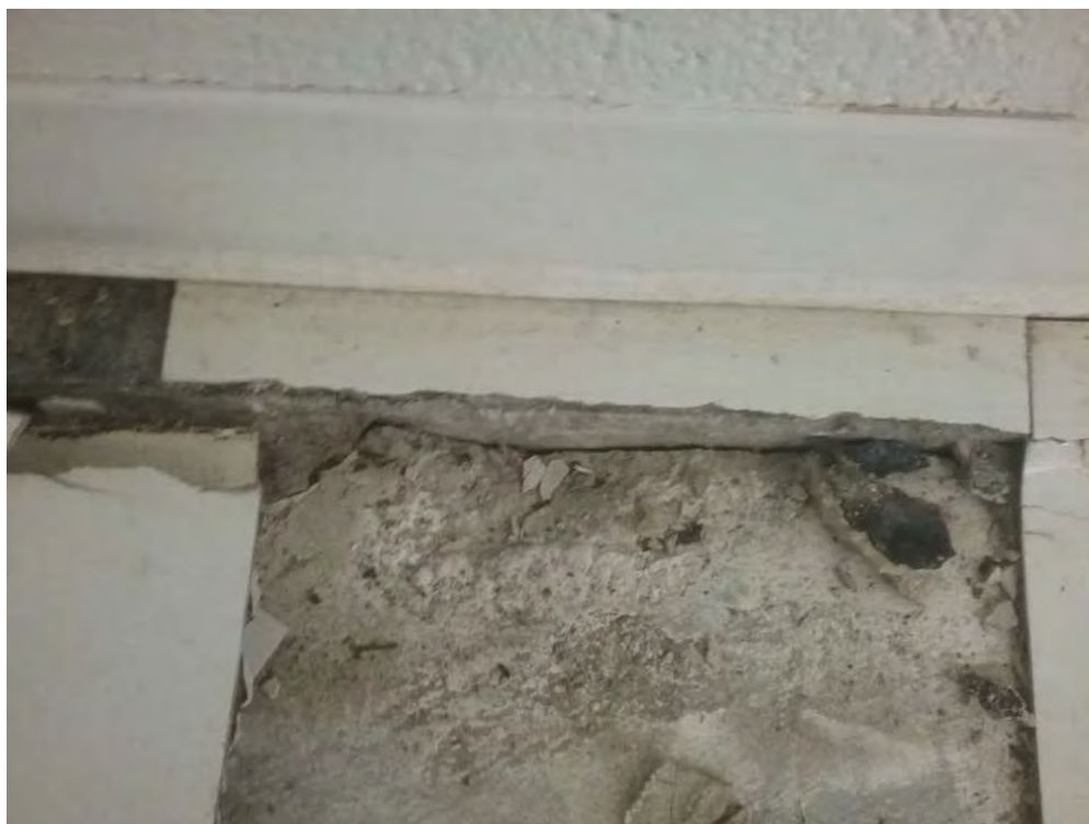
Photo 20 Depicting Close up of cracks observed in slab in Multi-Purpose Room
