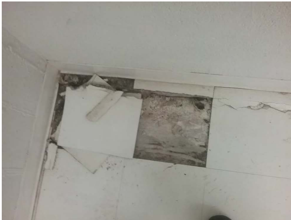
Photo 19 Depicting Broken and Raised Floor Tile in Multi-Purpose Room. (Note: Cracks observed in slab run entire span of wall on south side)
