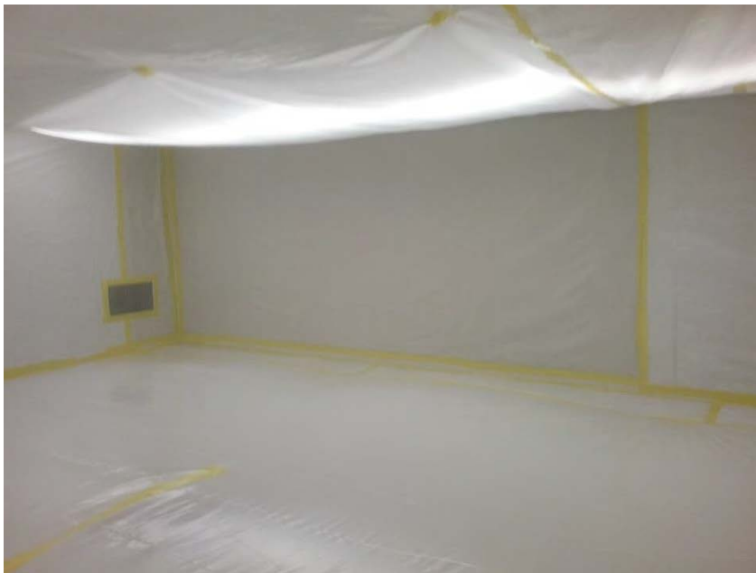
Photo 7 Depicting South Wall of Multipurpose Room following installation of enclosure isolating walls, ceiling and floor.
