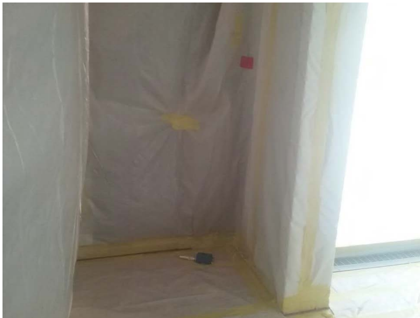
Photo 11 Depicting Wall Sample Apparatus in Intermediate South area following installation of enclosure isolating walls, ceiling and floor.
