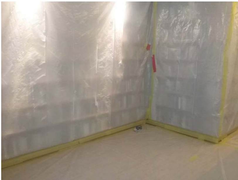
Photo 9 Depicting Intermediate South Wall following installation of enclosure isolating walls, ceiling and floor
