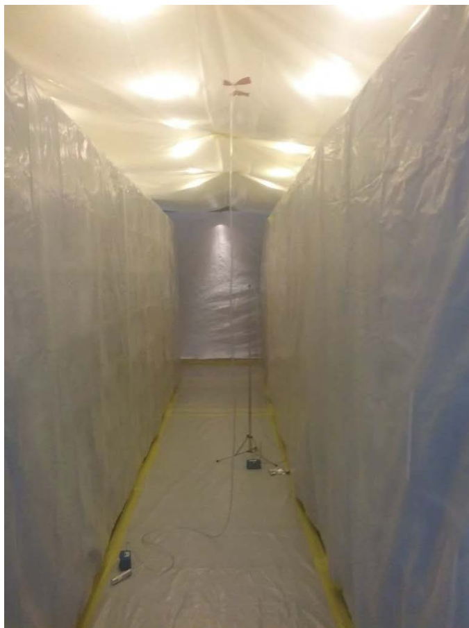
Photo 10 Depicting Ceiling and Ambient Sample Apparatus in Intermediate South area following installation of enclosure isolating walls, ceiling and floor.
