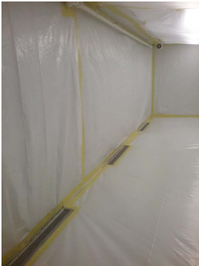
Photo 5 Depicting North wall of Multi-Purpose Room following installation of enclosure isolating walls, ceiling and floor.
