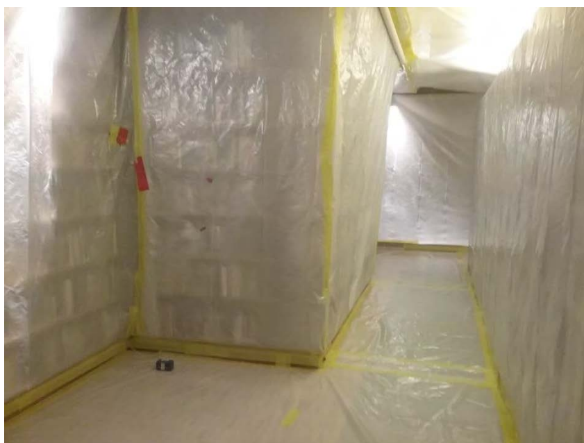
Photo 12 Depicting Wall Sample Apparatus in Intermediate South area following installation of enclosure isolating walls, ceiling and floor.
