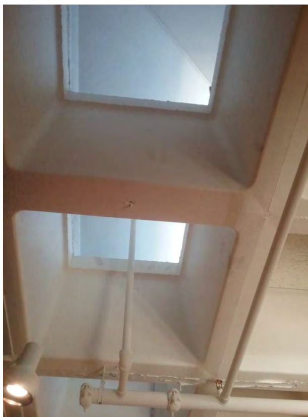
Photo 18 Depicting Ceiling Slab Opening in Intermediate South Room. Open to Space Above. Space represented by Ceiling Indoor Air Sample.
