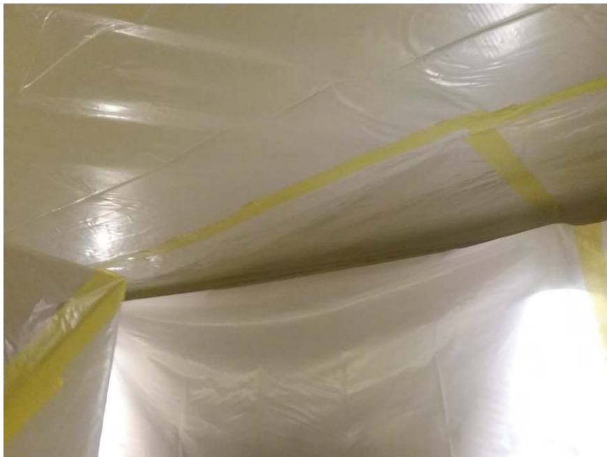
Photo 13 Depicting Close up of separation of wall and ceiling in Intermediate South area following installation of enclosure isolating walls, ceiling and floor.
