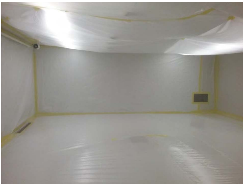
Photo 6 Depicting East Wall of Multipurpose Room following installation of enclosure isolating walls, ceiling and floor.
