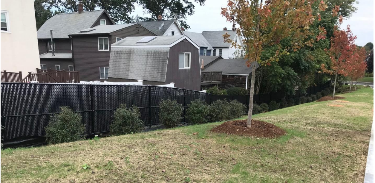
Privacy Fence installed along property line – 10/2/19
