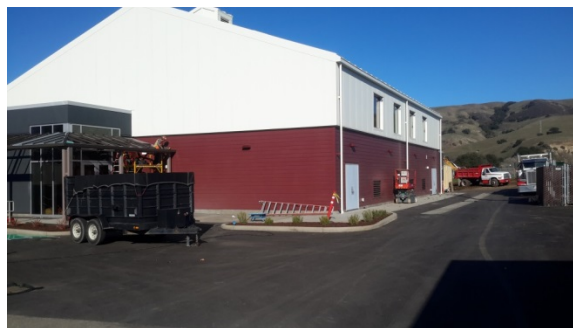
Charter School of Morgan Hill – Multipurpose Room Progress
