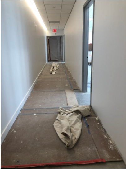
Construction in the old Business Office suite, creating a new classroom.
