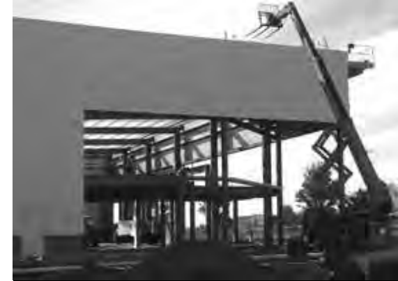
Trevisan USA built a new 17,000 square foot structure on South Street.
