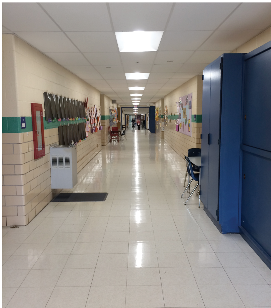
Drinking fountains protruding into Corridors more than allowed by ADA. Need to verify if storage cabinets protrude more than 4" into corridor exiting.
