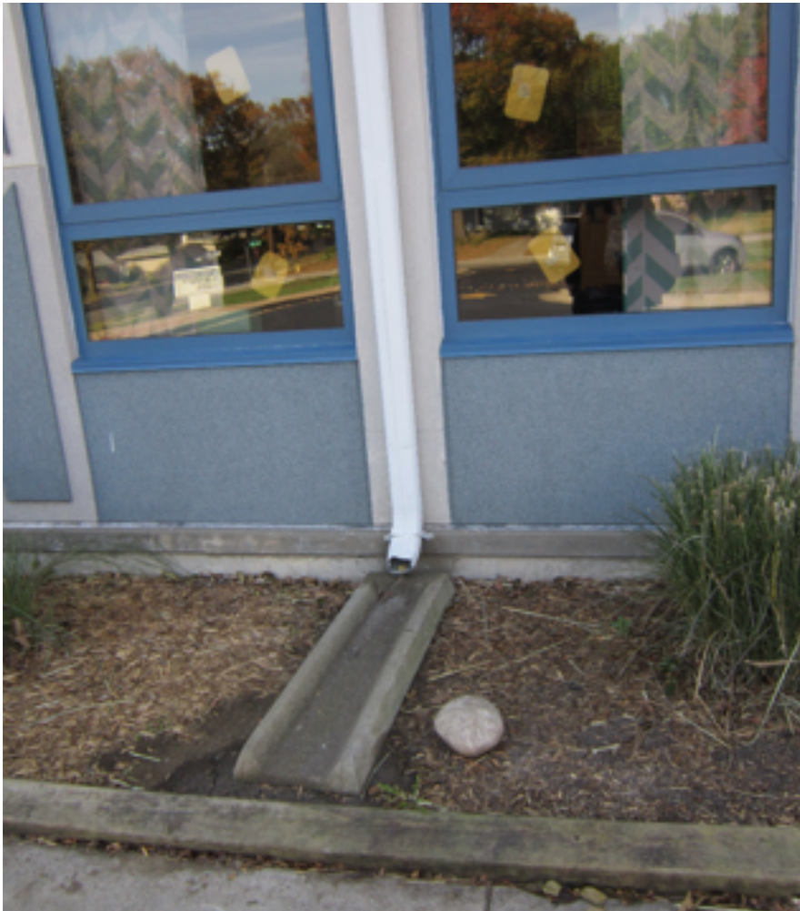
Roof drainage discharge on sidewalk
