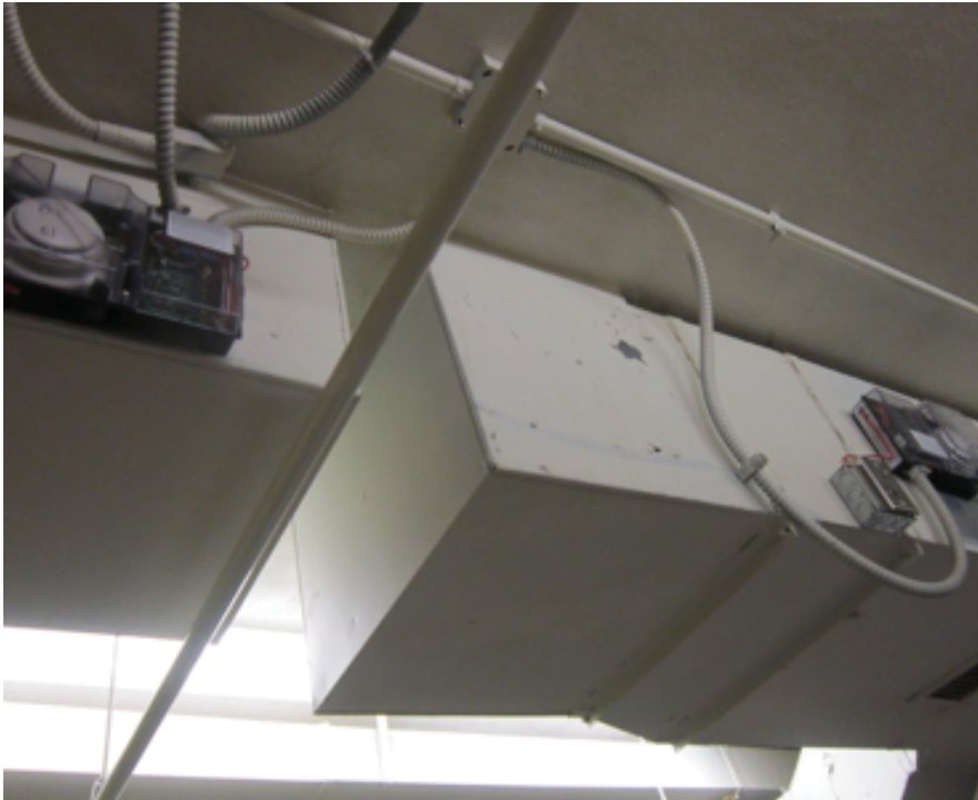
Smoke Detection on HVAC equipment
