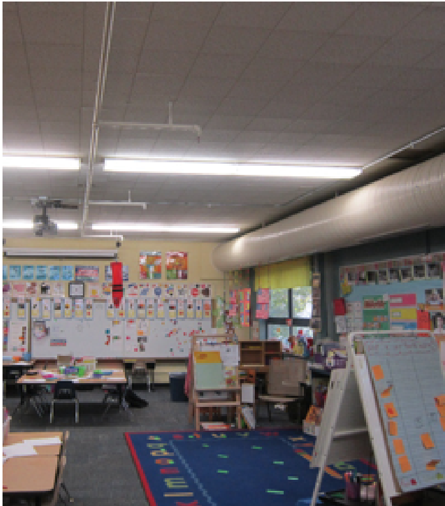
Exposed ductwork and sprinkler system in classroom space
