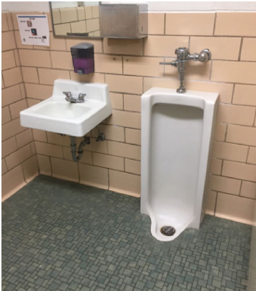
Floor mounted plumbing fixtures
