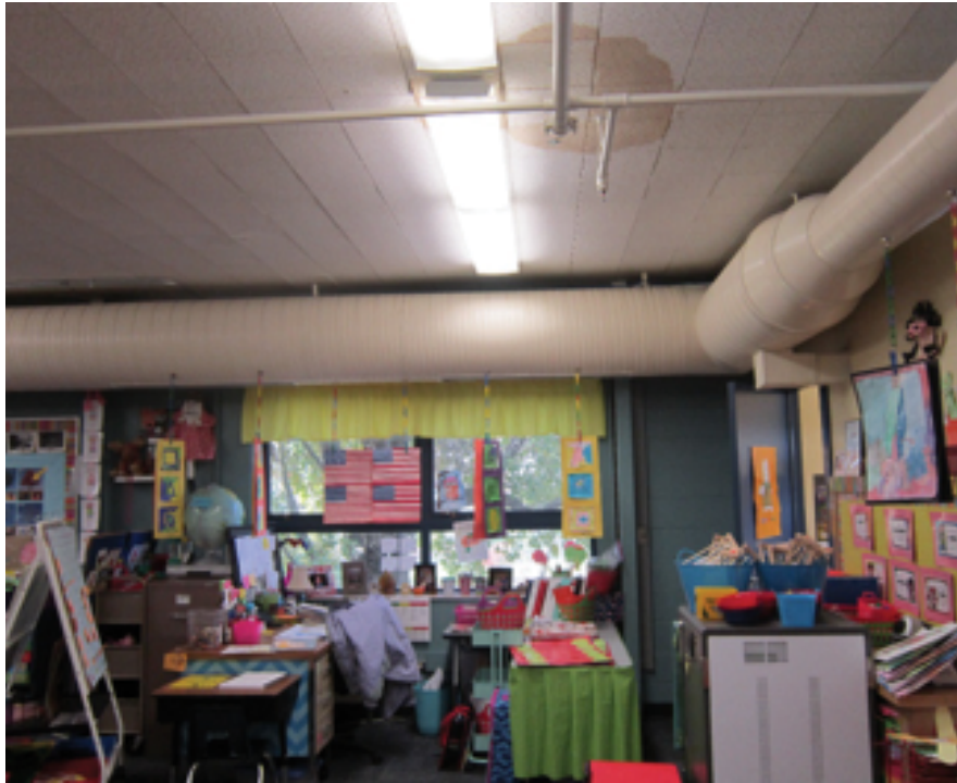
Ductwork exposed in classroom & ceiling water damage
