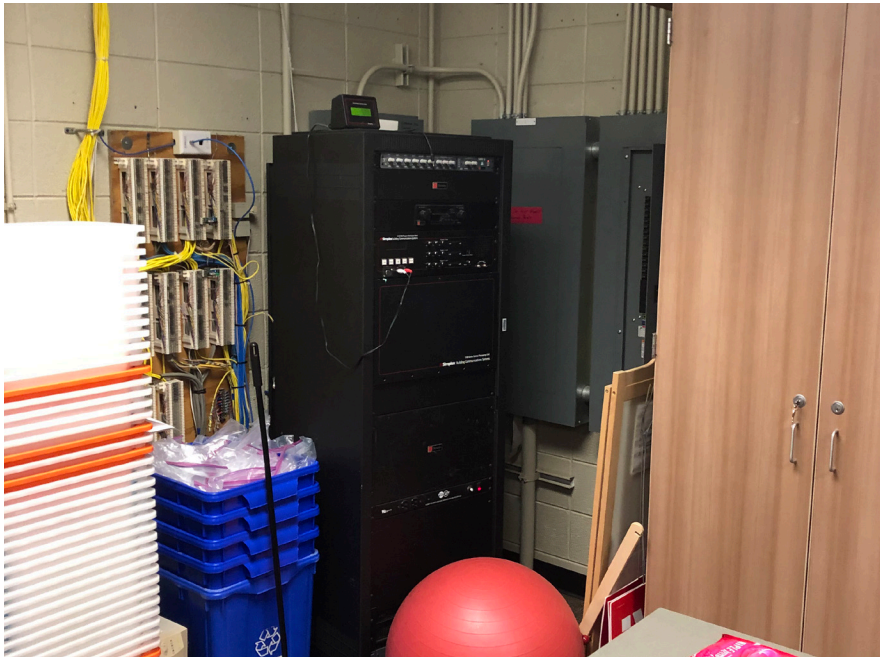
Data rack and electrical panels located in workroom Electrical panel does not have code-required clearance.
