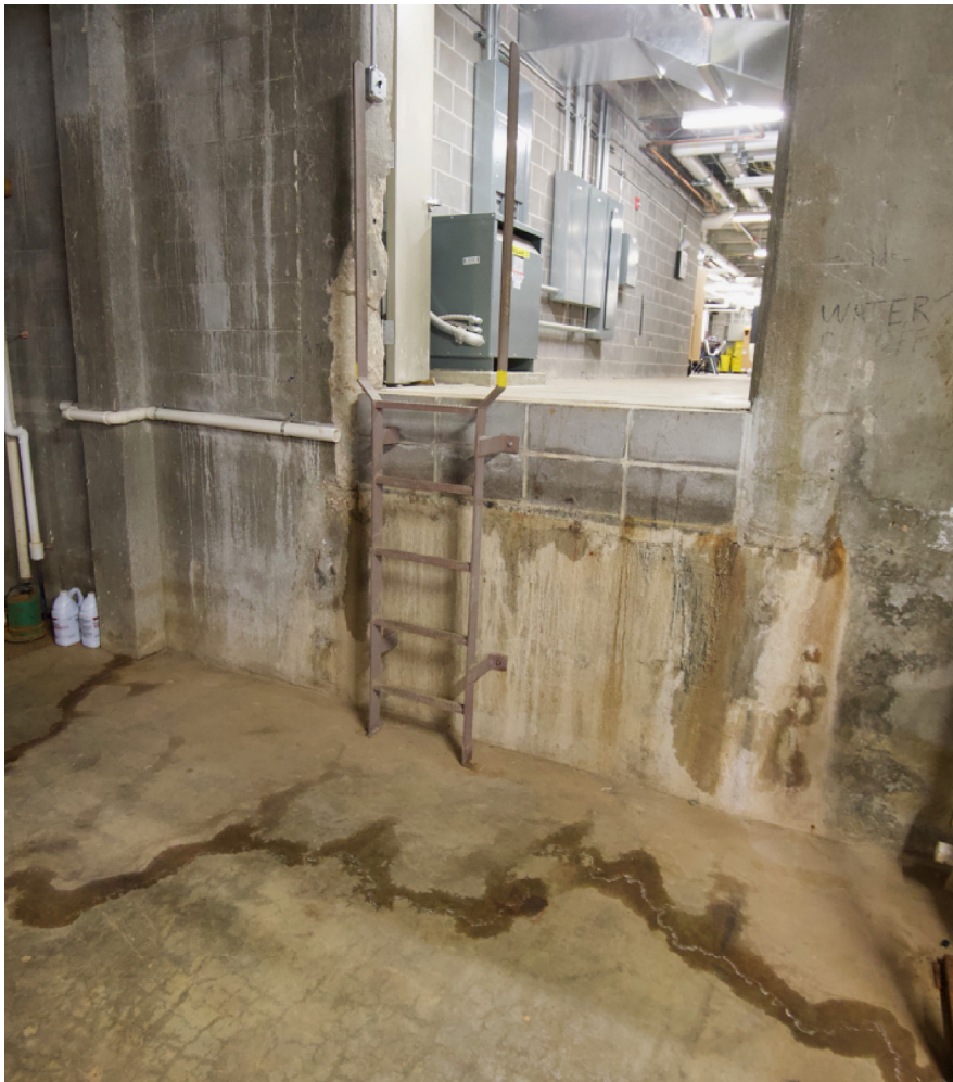
Lower mechanical room floor can take on water periodically.
