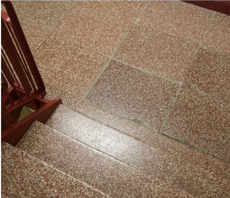
Mismatched floor patching in stair tower.
