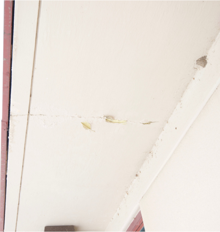
Cracks in exterior soffit.
