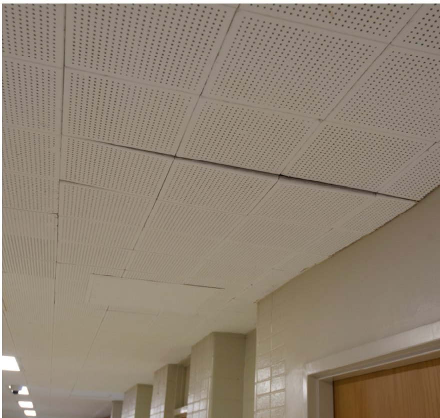
Locations where surface-mounted or glued ceilings are used require attention or replacement.
