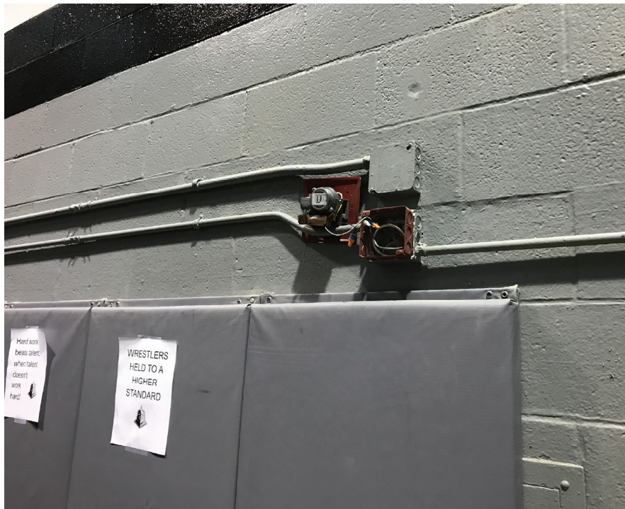
Open electrical J-box in the wrestling room.
