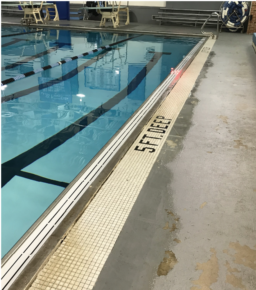
Pool deck need surfacing and upgraded tile.
