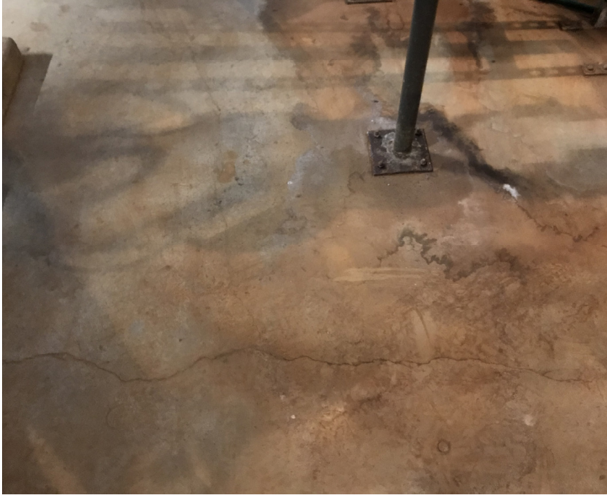
Evidence of basement flooding and concrete slab cracking in mechanical space
