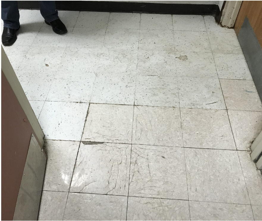
Damaged and cracked VCT evident
