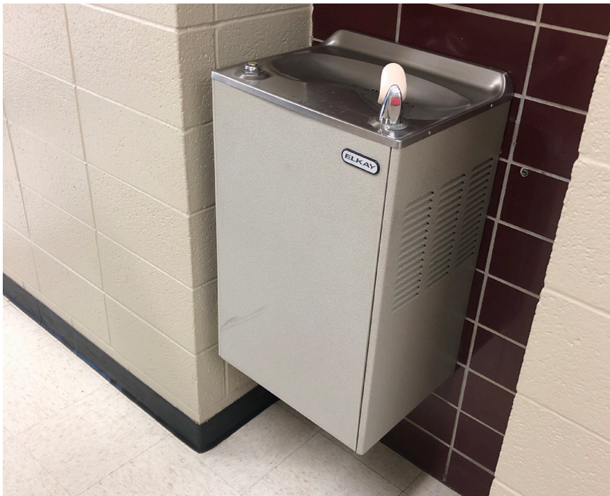
Water cooler does not meet ADA requirements and has no bottle filling station
