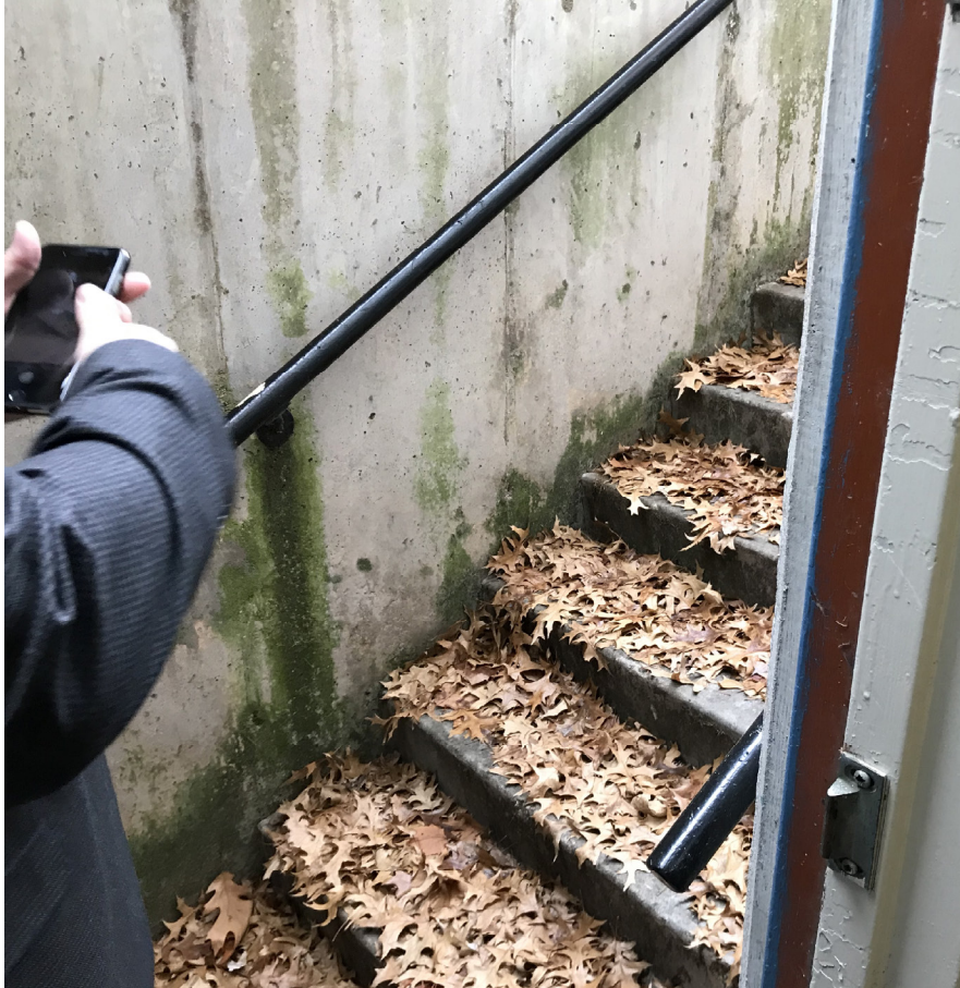
Exterior stair to basement has apparent drainage and mold issues
