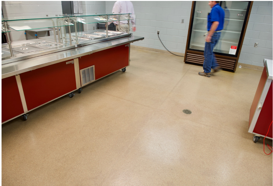
Kitchen floor is in good shape, but controls joints do telegraph through and should be monitored for potential failure in the future.
