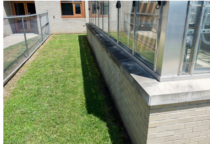
Some staining of the cast stone on the north elevation of the greenhouse.
