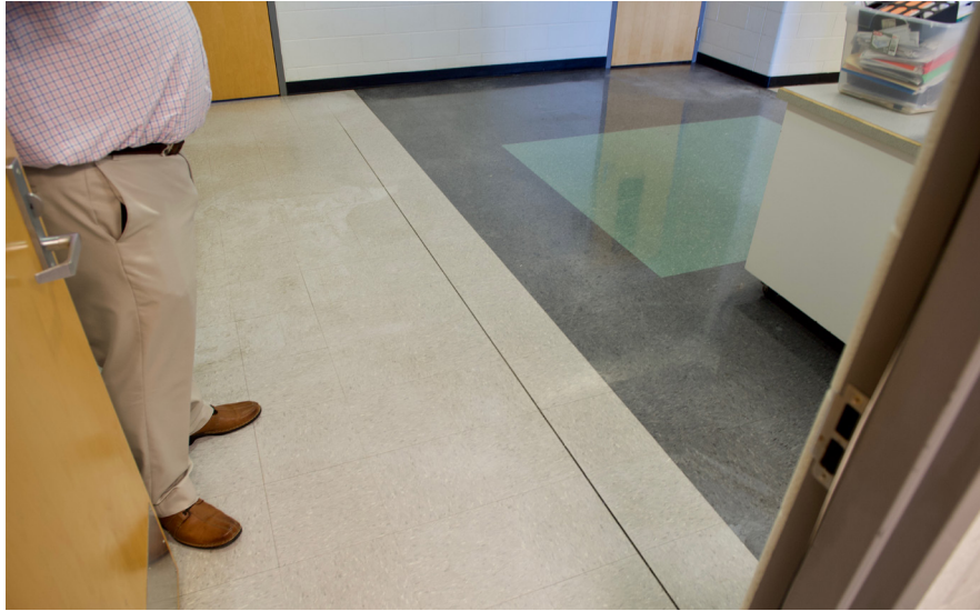
Separation in the floor tiles in this location may indicate movement in the structure or an expansion joint.
