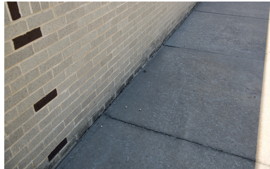
Some staining at the lowest brick along the sidewalk outside the common space.
