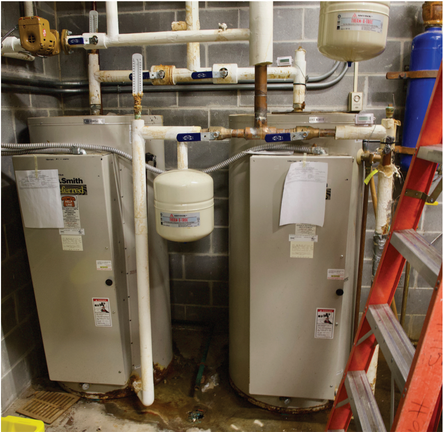
Boilers are in decent shape but may be nearing end of life in the next decade.
