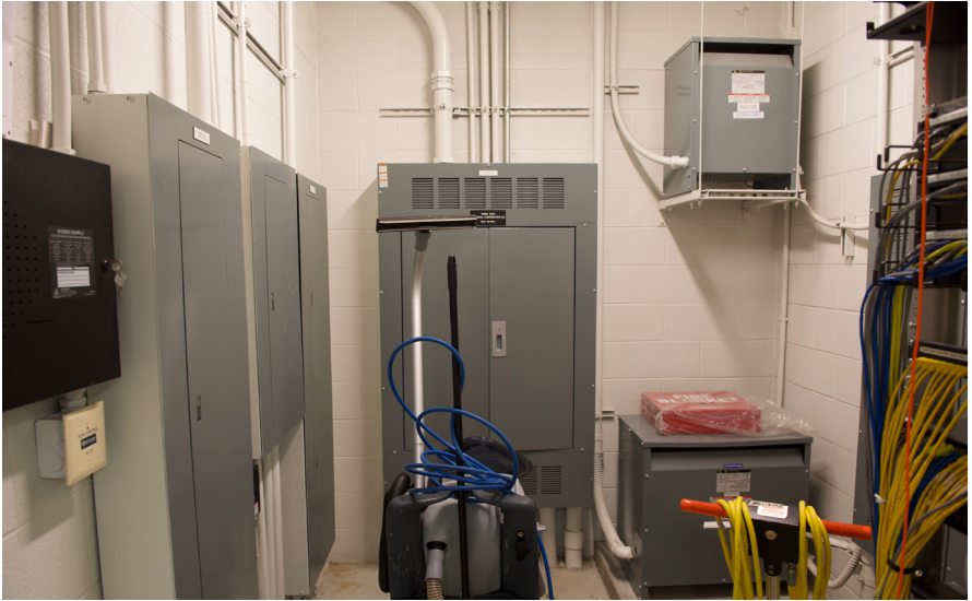
Electrical and Data share same room, no security for data.
