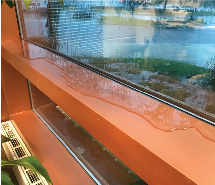
Projection windows have been a constant leaking issue.
