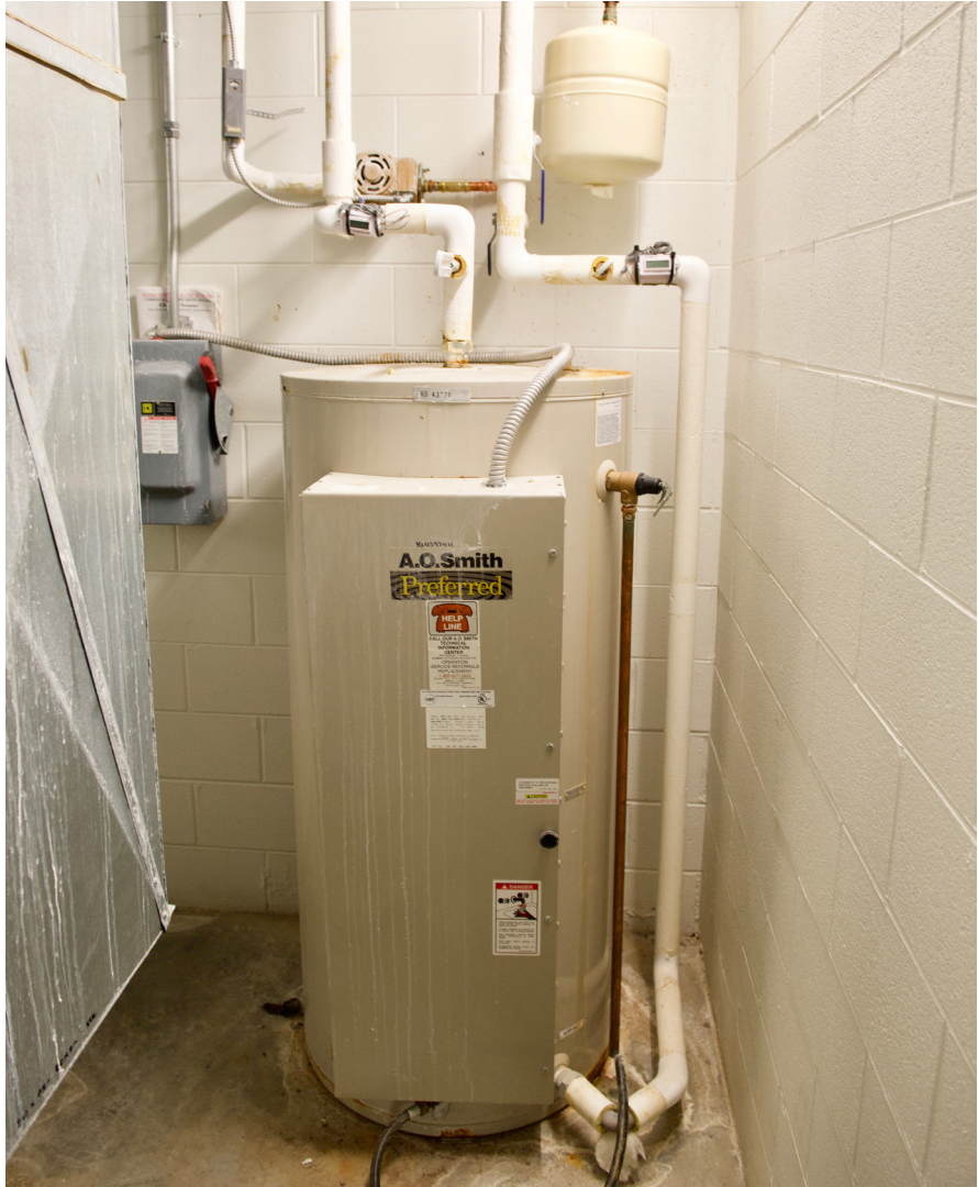
Hot water tanks may be nearing end of life.
