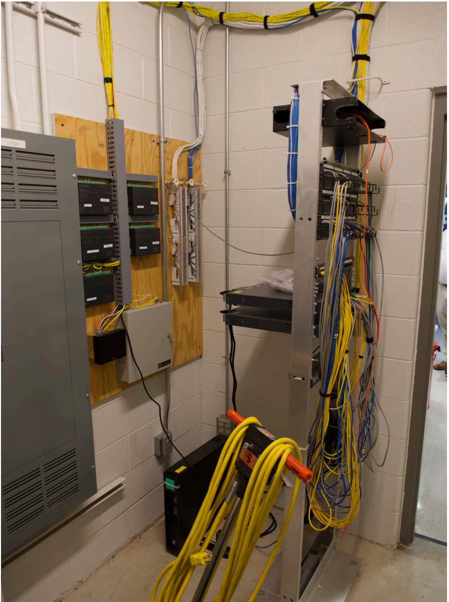
Data Rack and Phone patch board.
