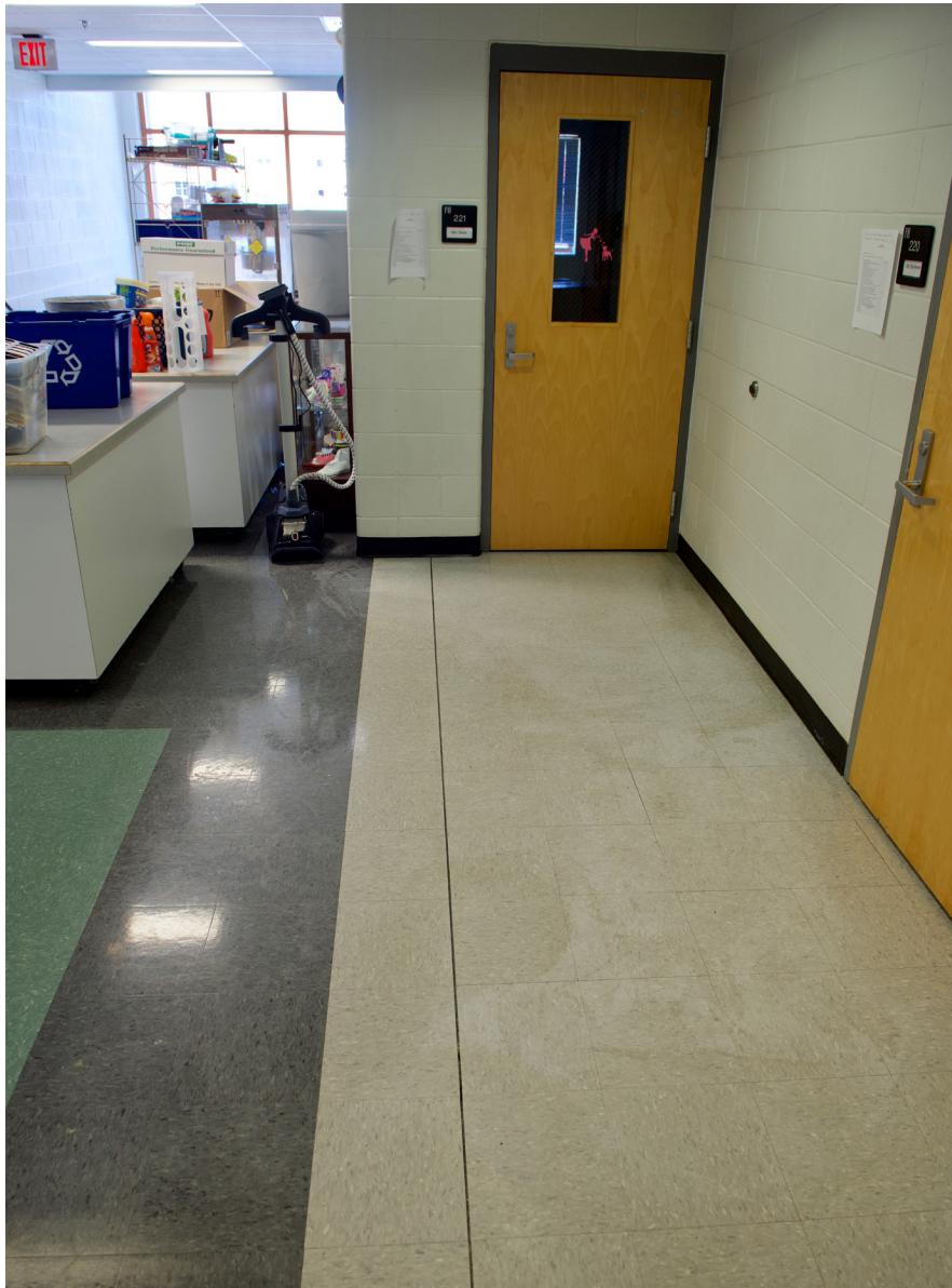
Separation in the floor tiles in this location may indicate movement in the structure or an expansion joint.
