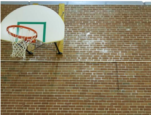
Efflorescence in gym
