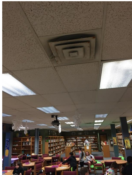
Supply diffuser rusting due to high humidity levels.
