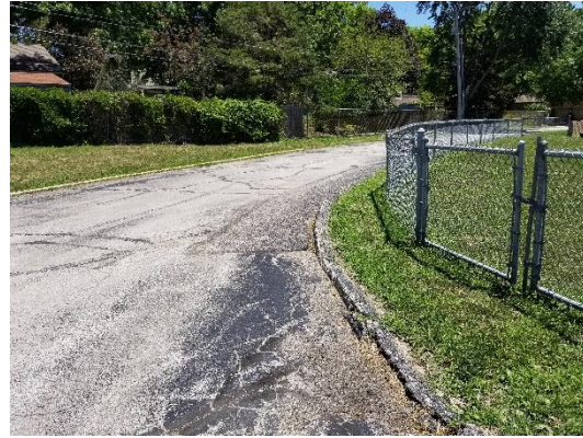
Deteriorated asphalt and curbing
