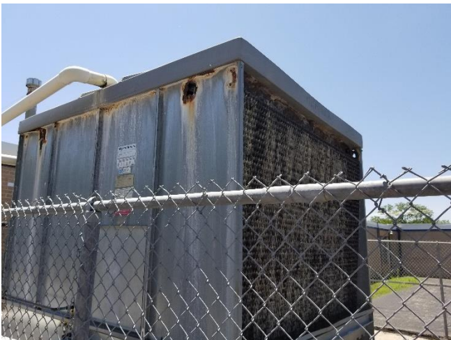
Chiller in need of significant repairs or replacement
