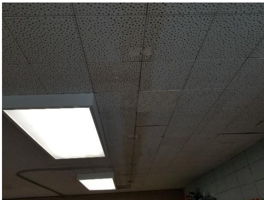
Water Damaged ceilings
