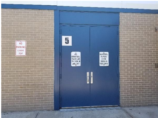
Exterior Hollow Metal Doors
