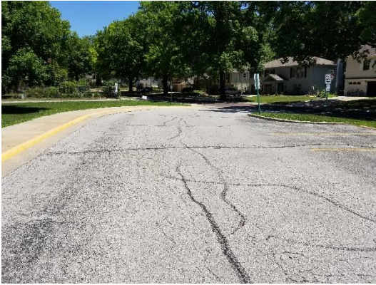
Alligatoring Asphalt
