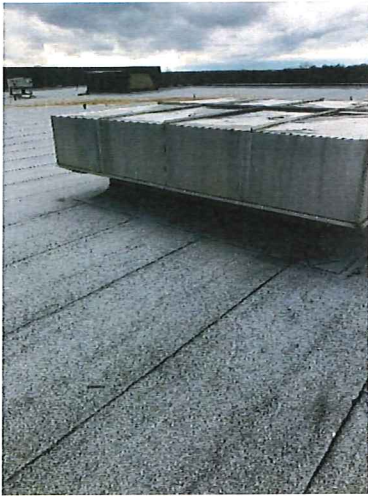
Leaking Roof Hood
