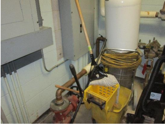
Water service installed in required clearance of panelboard.
