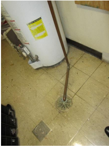
Water heater & drain in same closet as Data Rack.
