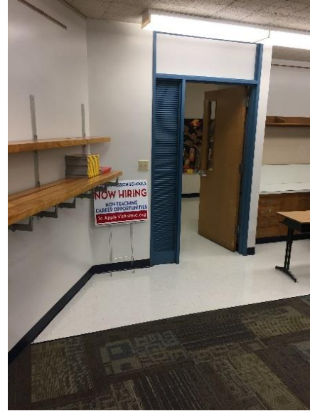
Return air transfer from classroom to corridor.
