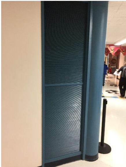
Corridor being used as return air path.
