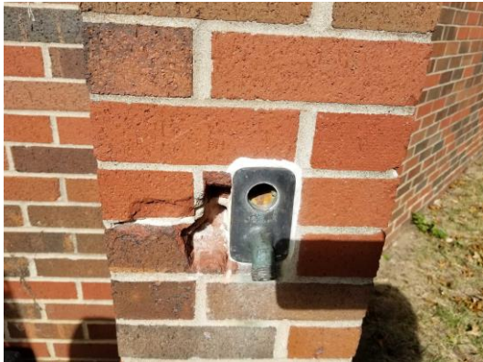
Damaged Brick at old hose bib
