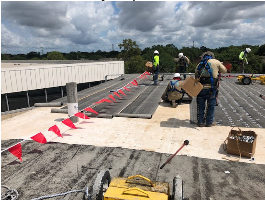
Installation of new roofing overlay continues.
