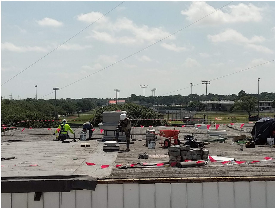
Installation of new roofing overlay continues.
