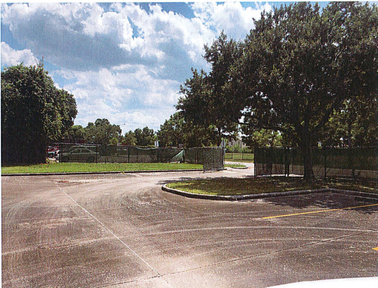
Construction fencing in place
