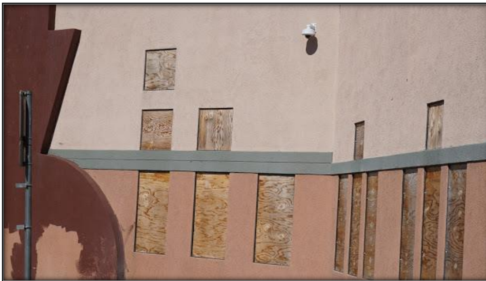
Figure 5: Work remains at the Mathson multipurpose building
