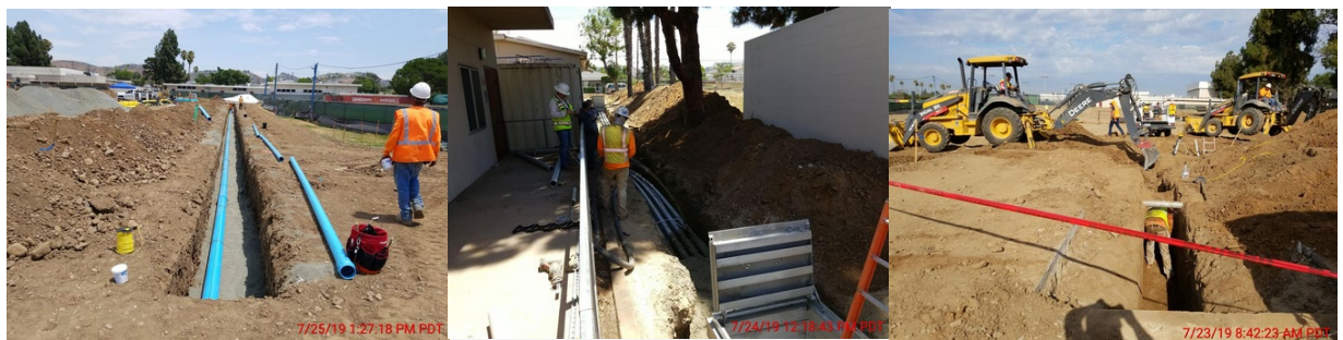
General Contractor, Angeles Contractor, excavating, placing and uncovering underground pipes, setting trench, and slurry in new underground conduit lines.
