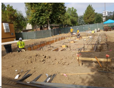
General Contractor, Swinerton Builders, excavating, placing the interim kitchen modular forms for concrete pad pour, and grading.
